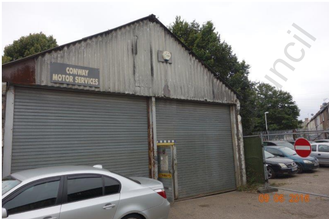
Corrugated workshop building
