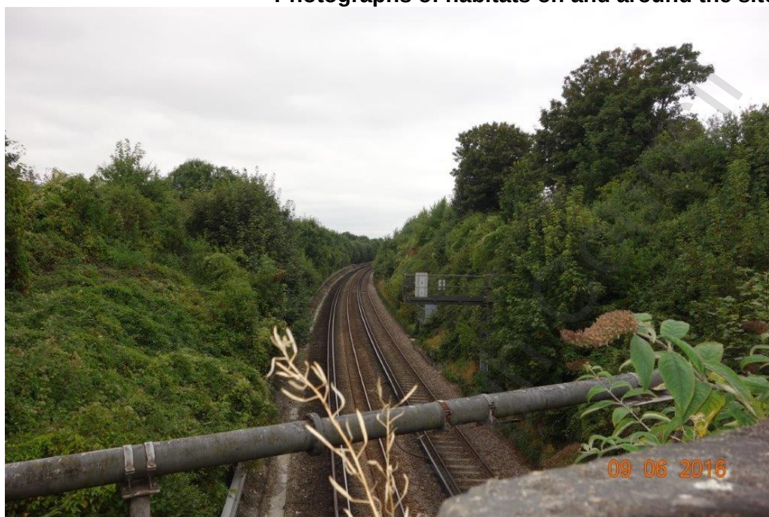
The site is the north (right) of the sunken railway line (looking west)
