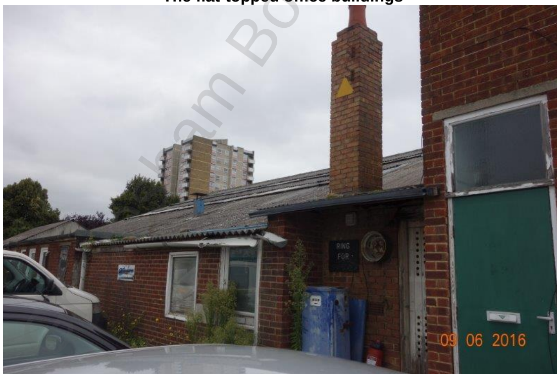
An older part of the buildings with chimney and corrugated hipped roof
