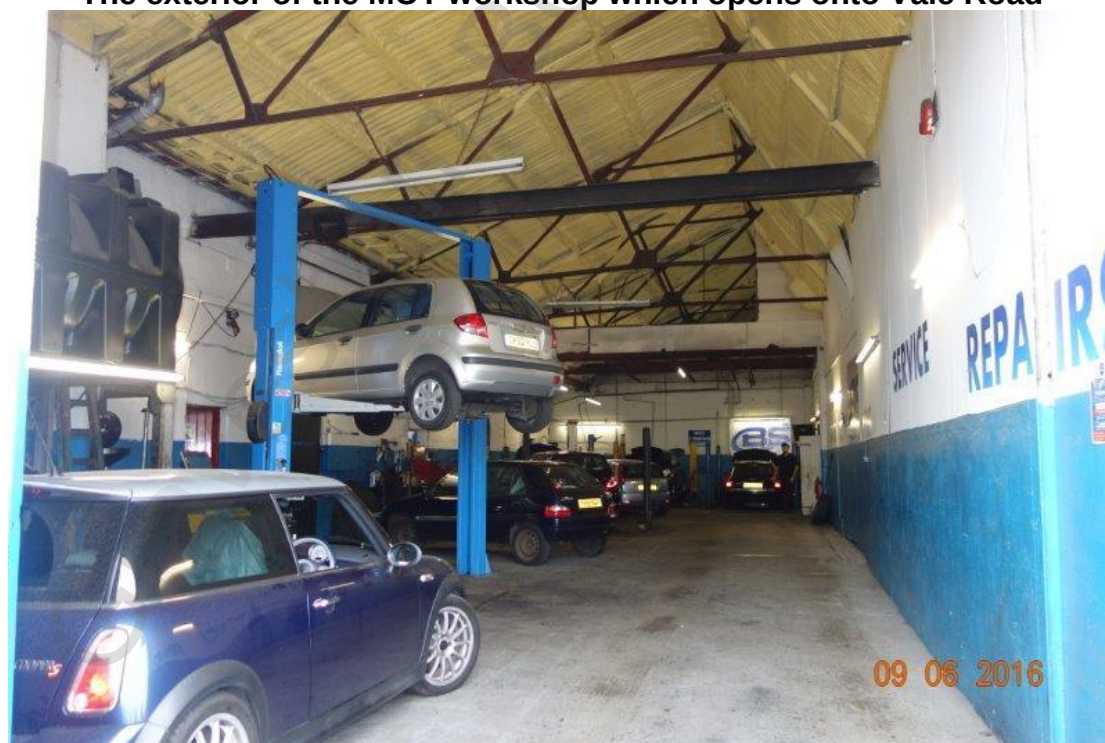
The interior showing the un-boarded roof
