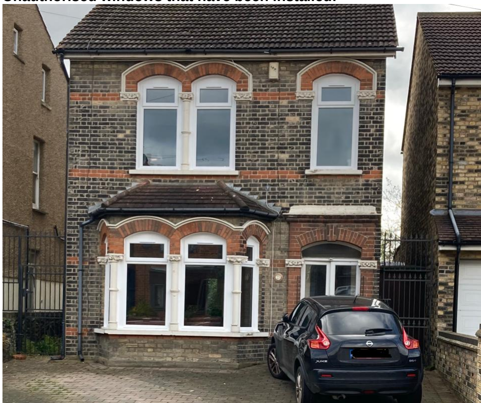
Unauthorised windows that have been installed:
