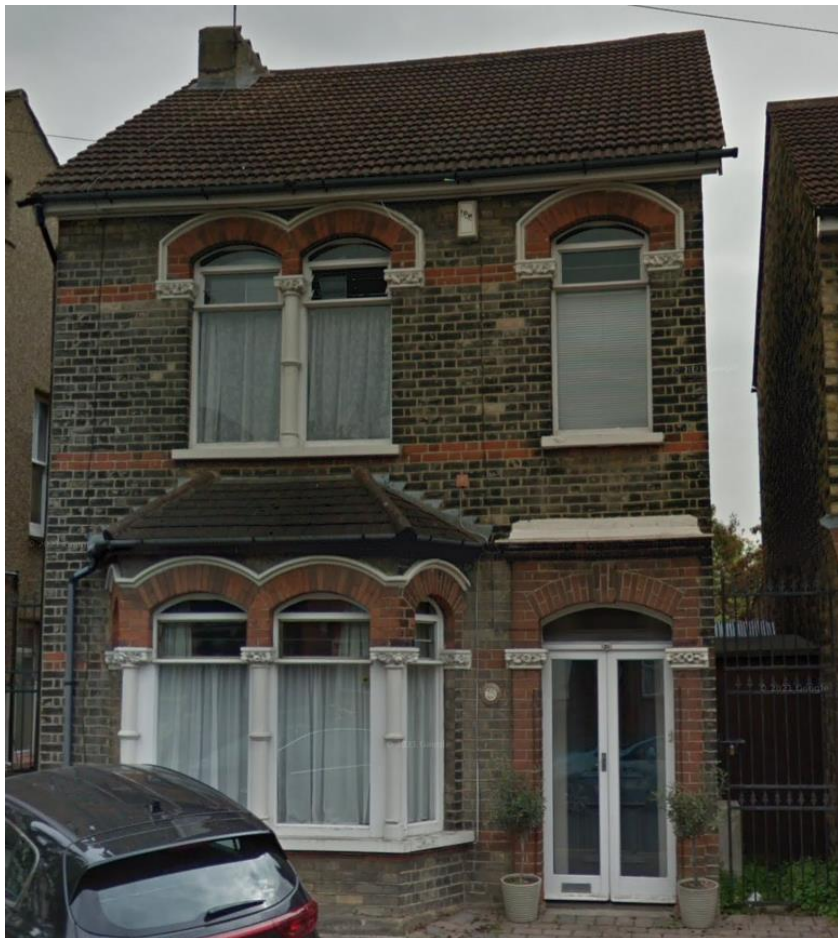
Previous windows which were removed:
