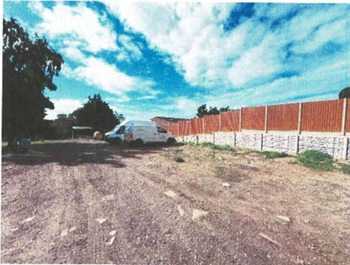
View of wall and fence along the west boundary.
