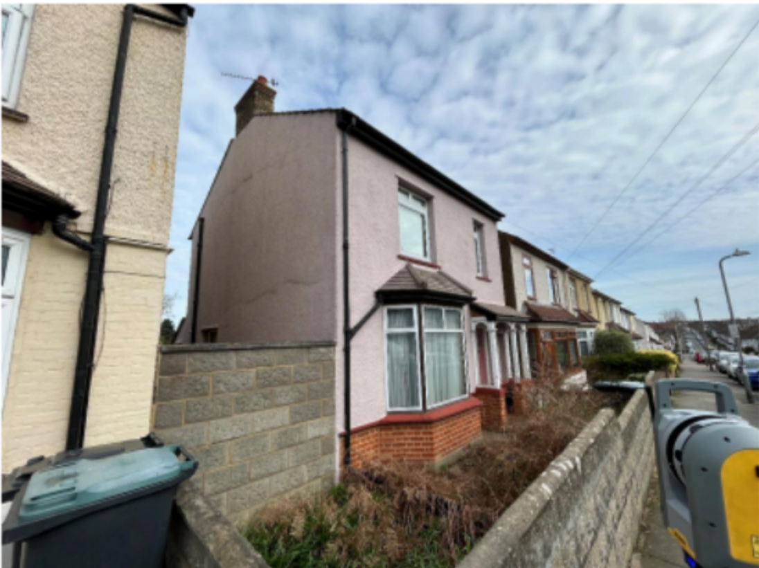
Photo 2. Front View – Park Avenue
