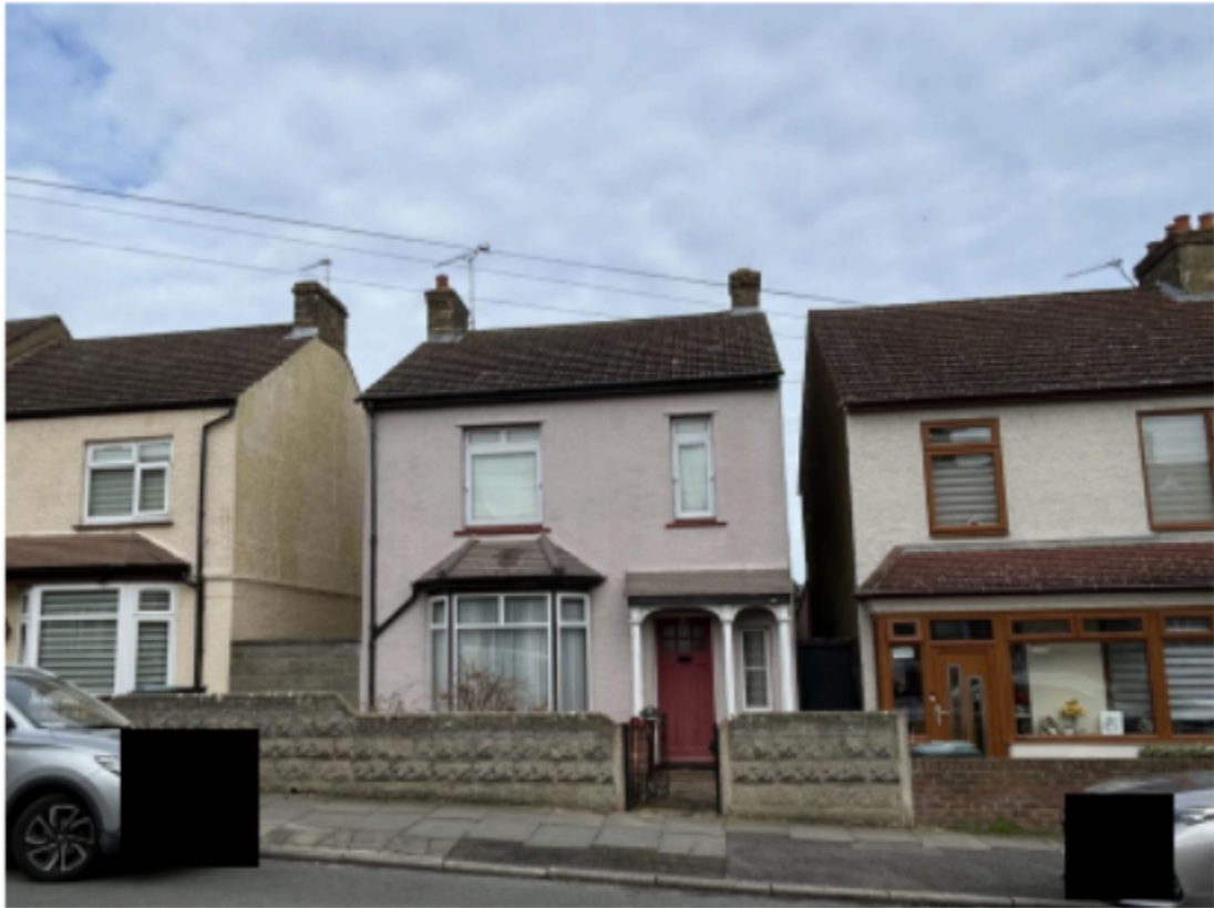
Photo 1. Front View – Park Avenue
