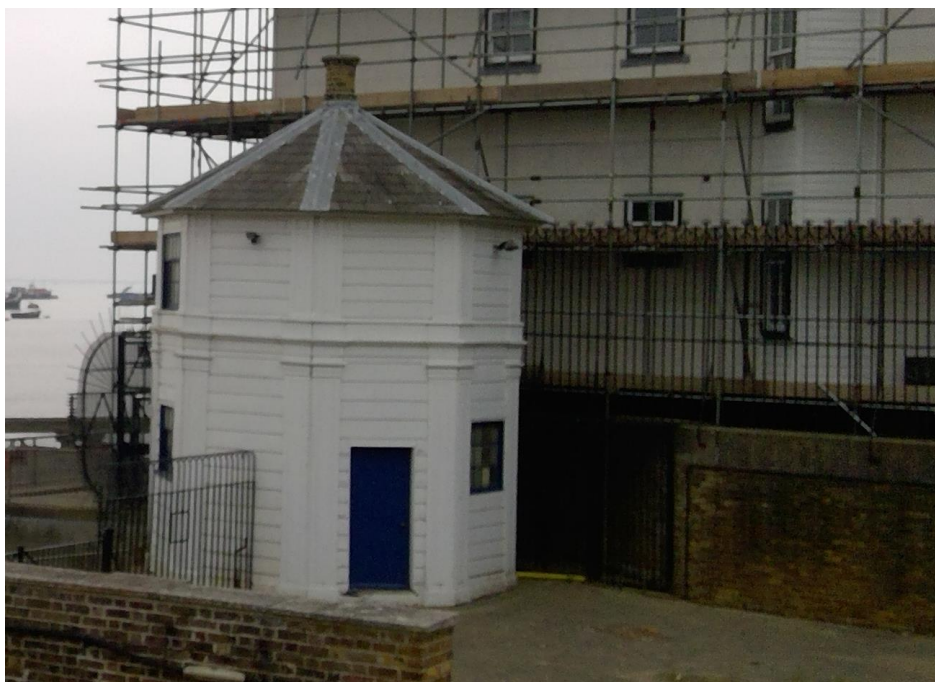
Gazebo and access from path to side of Heritage Quay as viewed from inside the site
