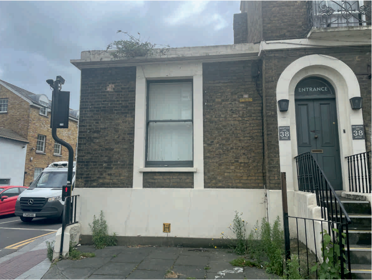
EXTERIOR - Front view from footway of Windmill Street showing single storey element to the side
