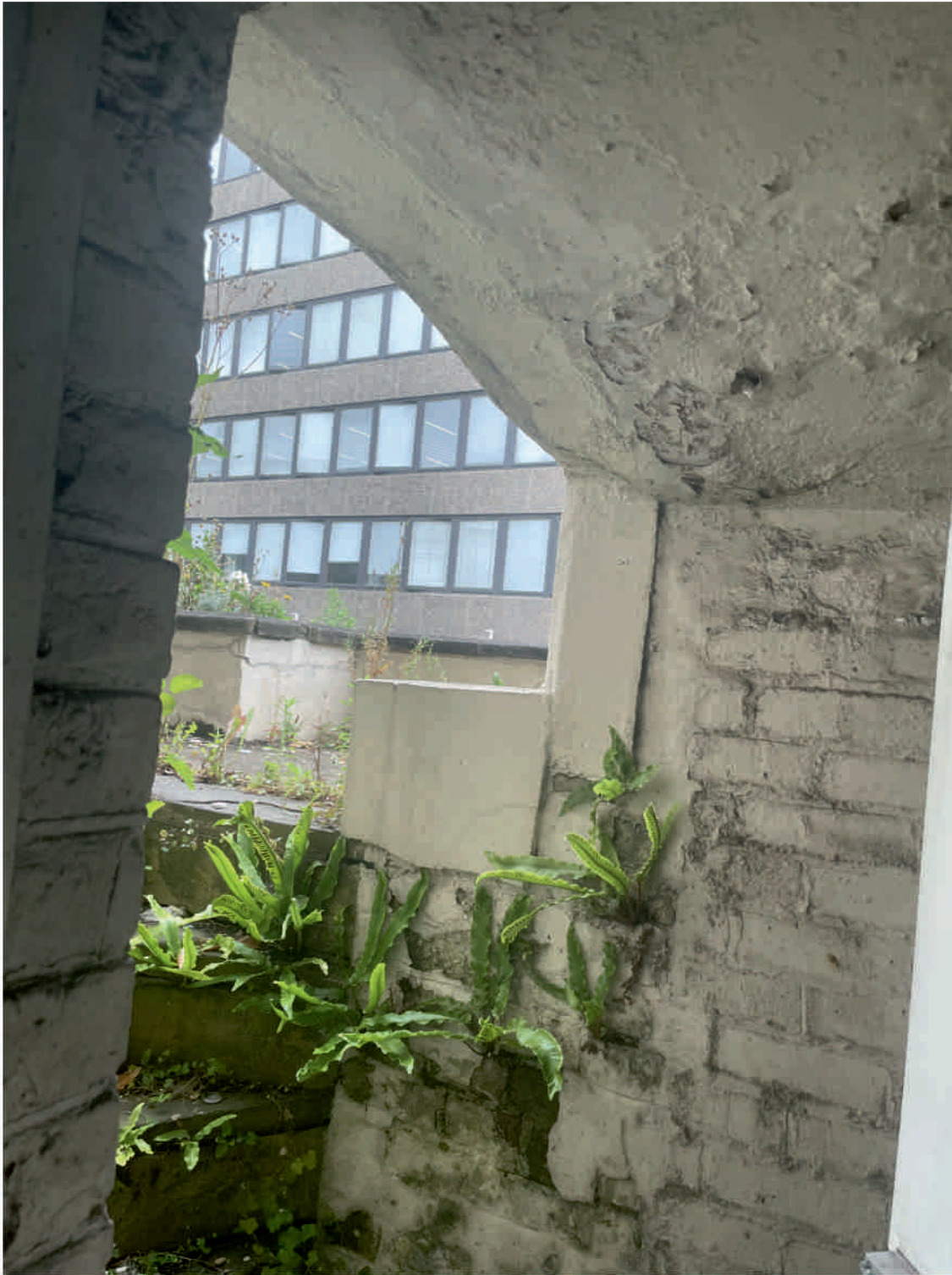
EXTERIOR - Top of basement stepst
