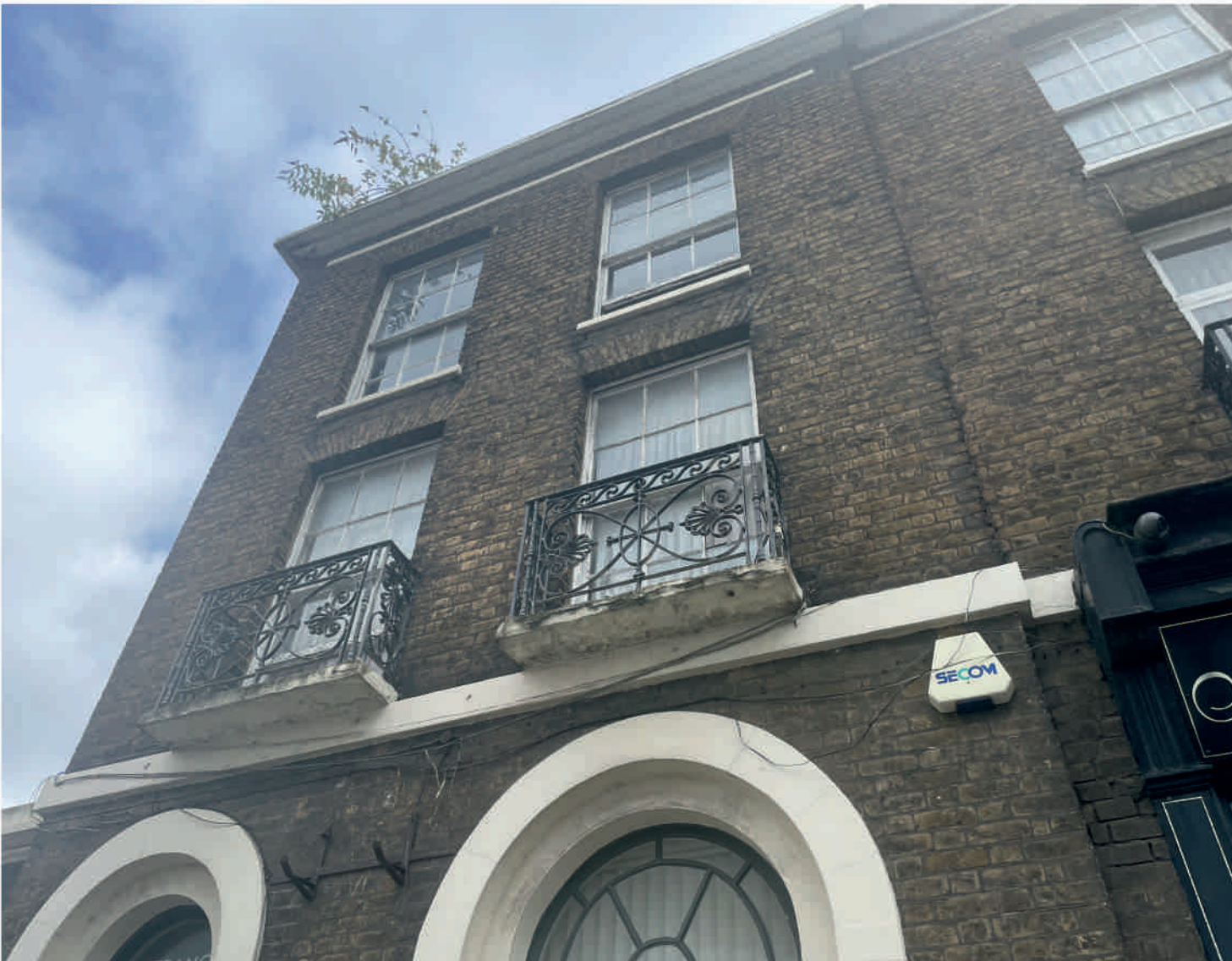
EXTERIOR - Detailed view of upper windows front
