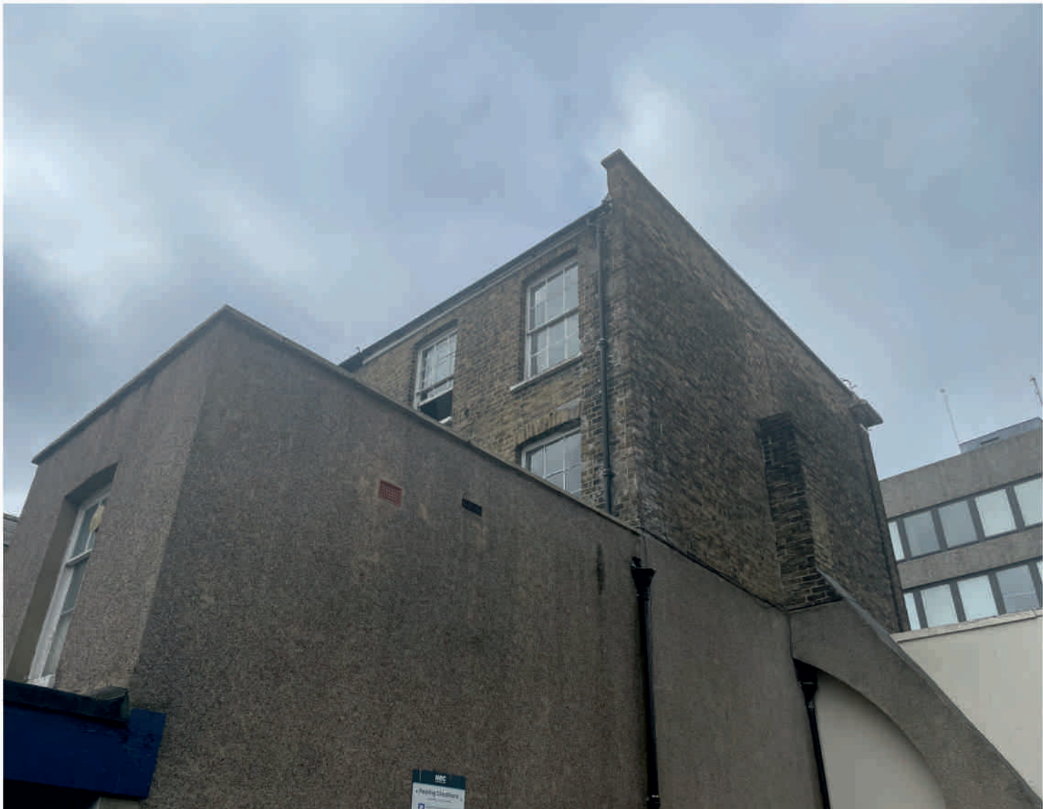
EXTERIOR - Detailed view upper side from Lord Street footway
