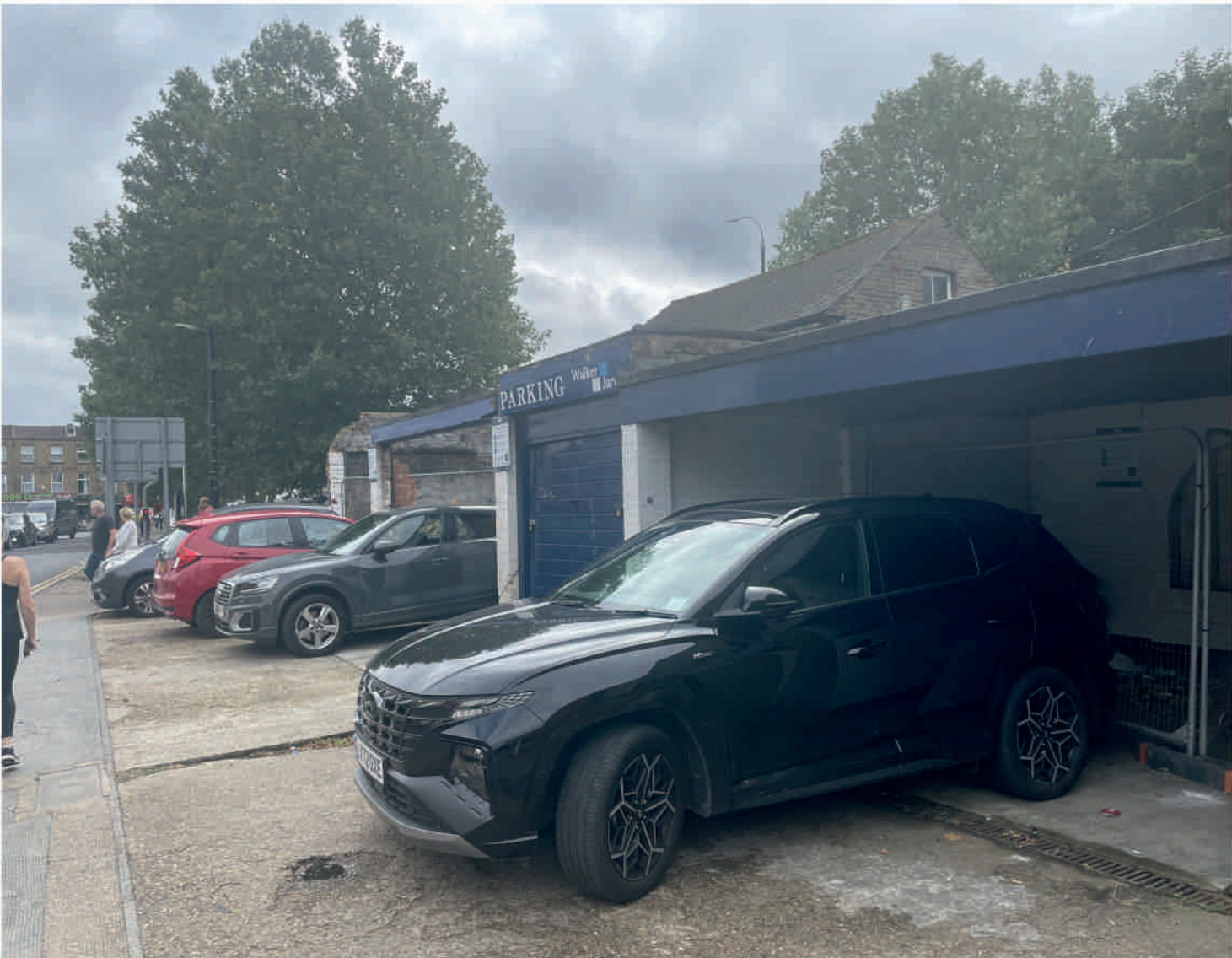
EXTERIOR - Lord Street existing parking forecourt
