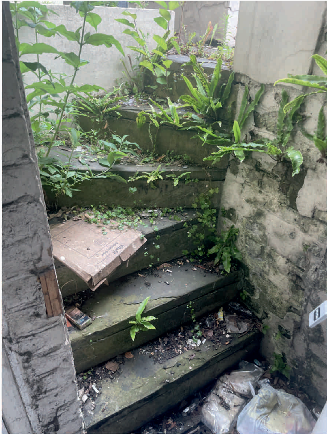
EXTERIOR - Basement steps below entrance stair
