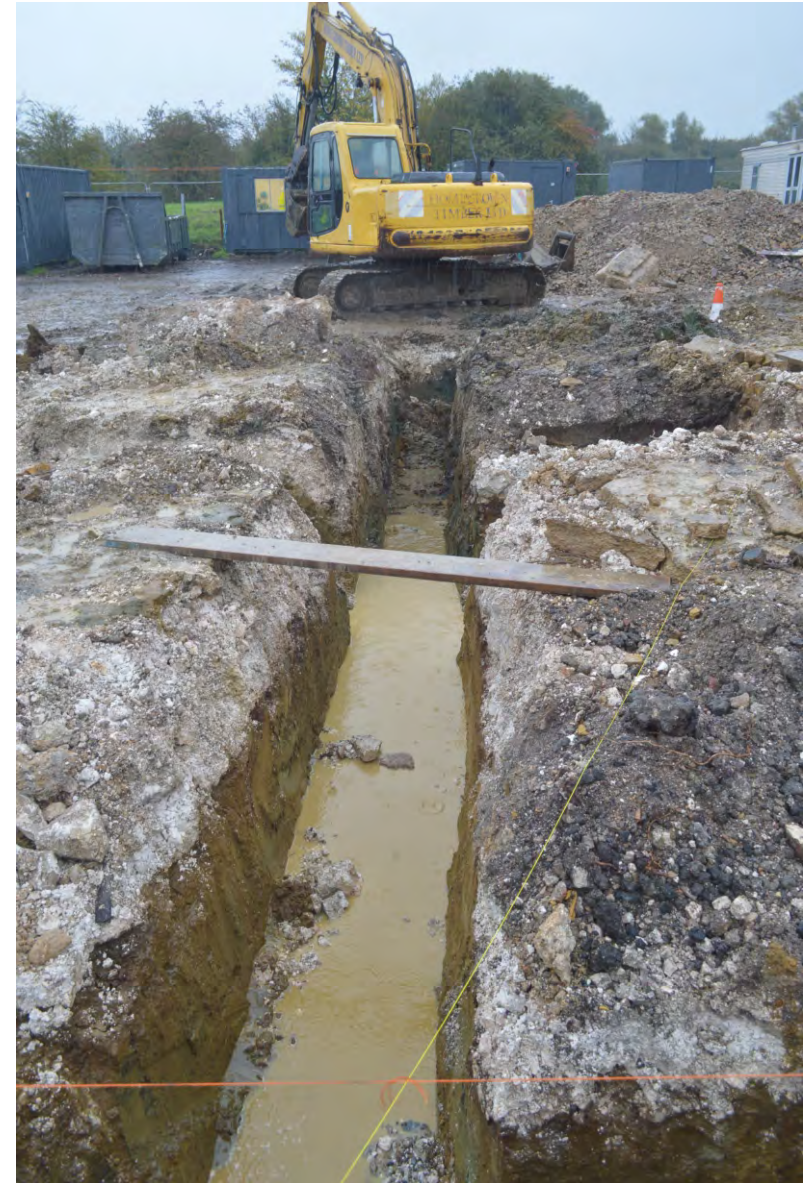
Plate 6. General view looking southeast along the line of the new open strip foundation trench.
