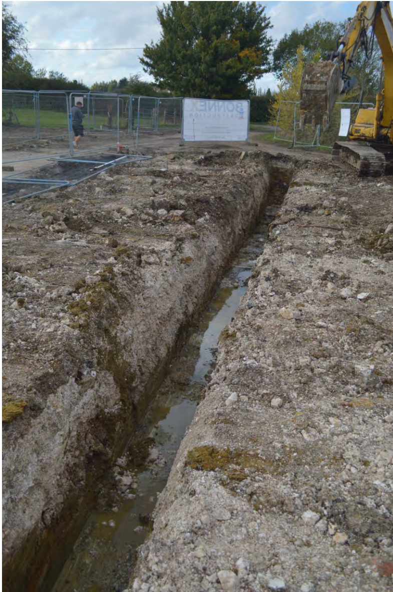
Plate 5. General view looking northwest along the line of the new open strip foundation trench.
