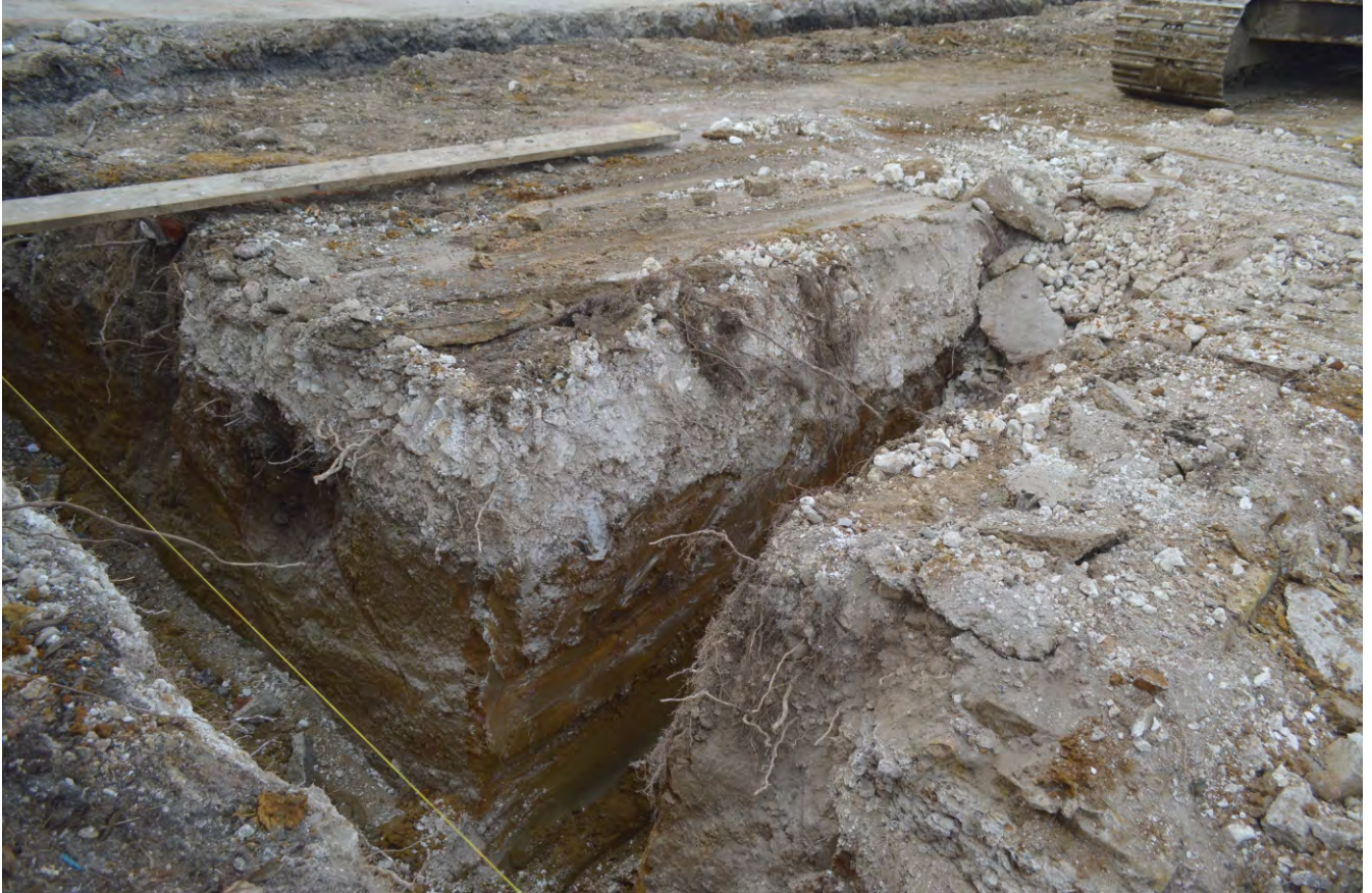
Plate 7. General view across the junction of new open strip foundation trenches showing natural bedrock geology sealed beneath compacted imported chalk and flint rubble dump deposit used to raise the local ground surface.
