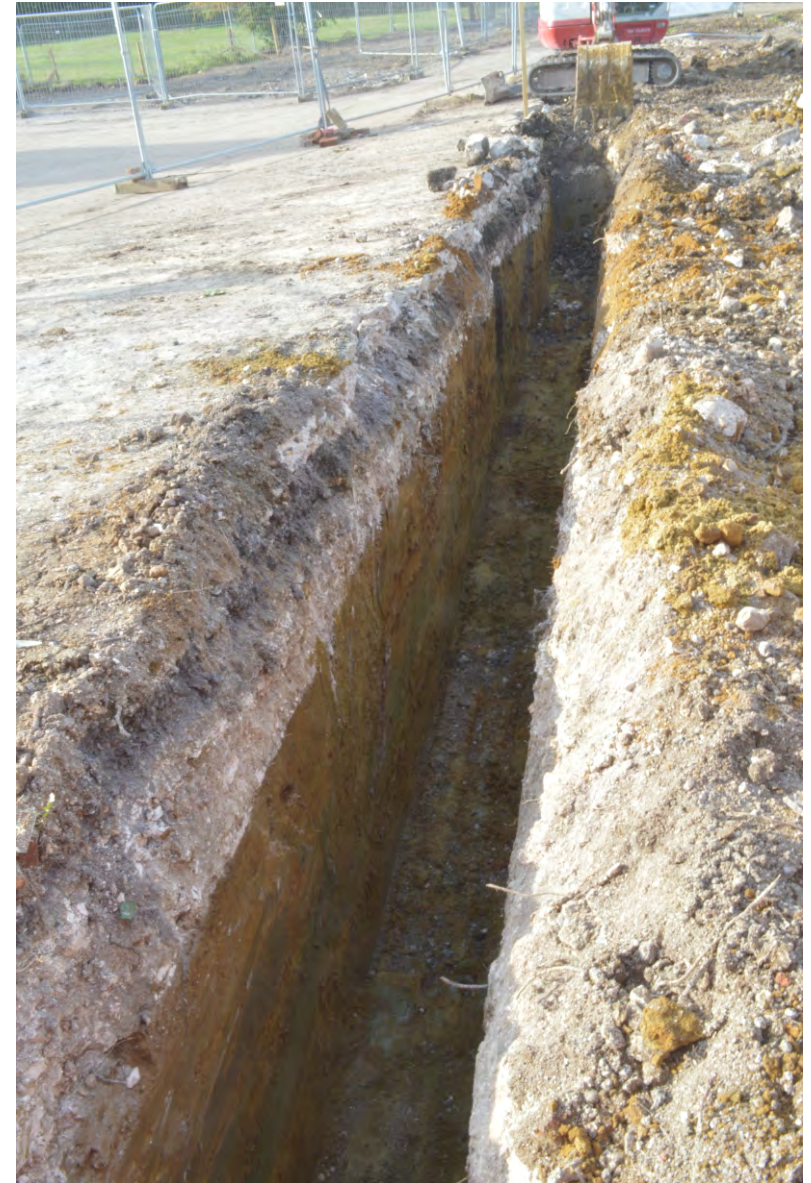
Plate 4. General view looking along the open strip foundation trench forming one main side to the proposed new building.
