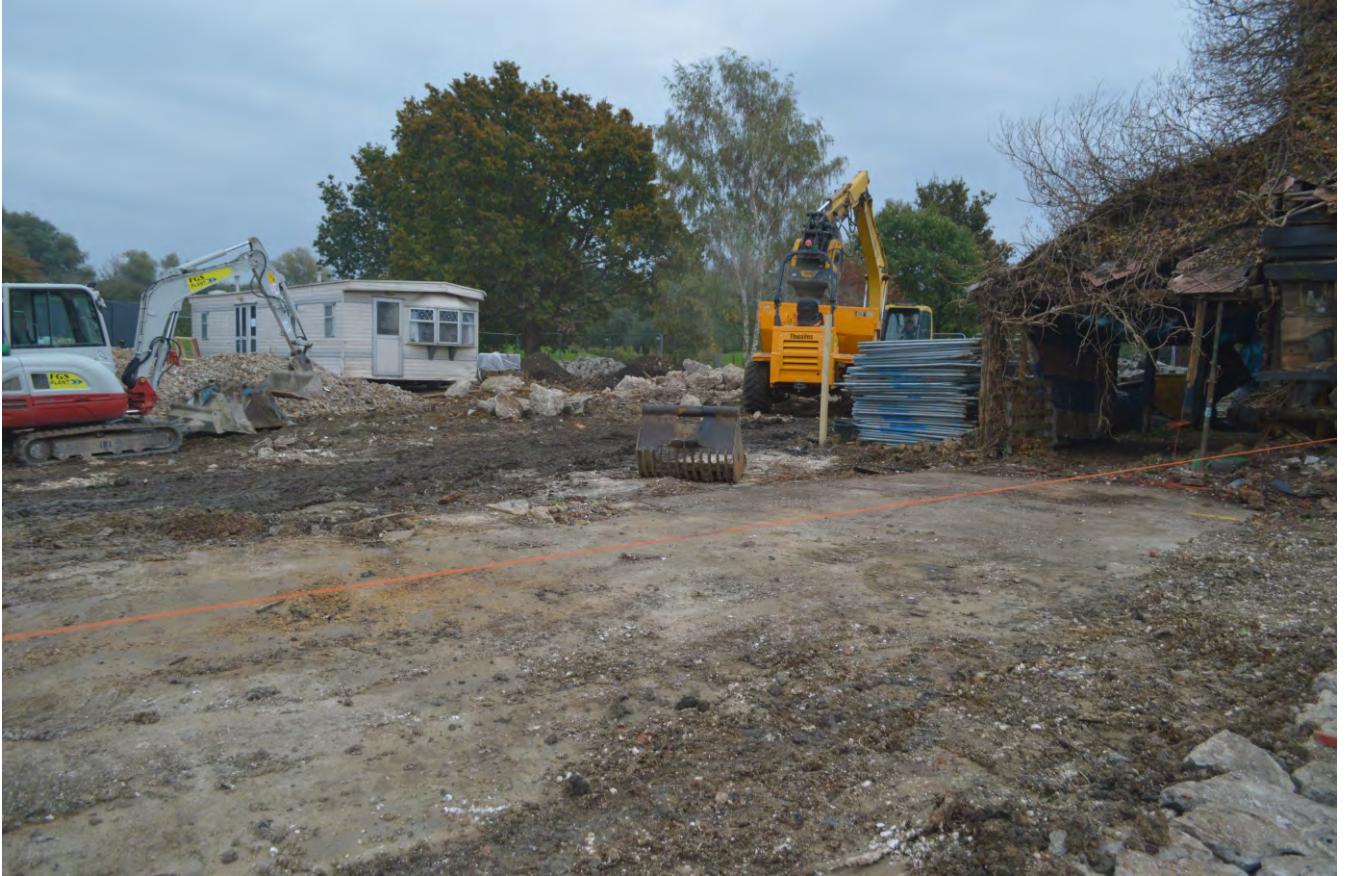
Plate 1. General view looking east across the proposed development site showing the northern end of the timber-framed barn (right) following clearance of the former farm building.
