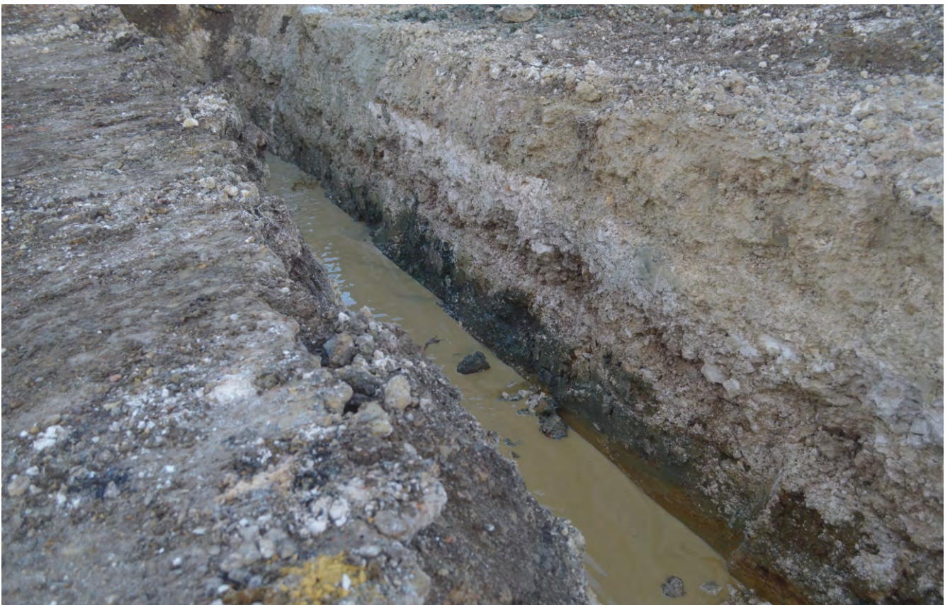
Plate 8. Section detail of the main open strip foundation trench showing darkened geology associated possible water feature sealed beneath imported chalk and flint rubble, itself sealed by further chalk rich dump deposit, all to raise the local ground surface.
