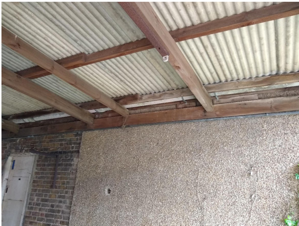
Photo 11 – Building C – roof.
