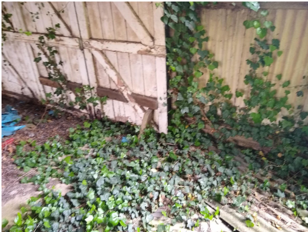
Photo 10 – Building C – sliding door to north wall.
