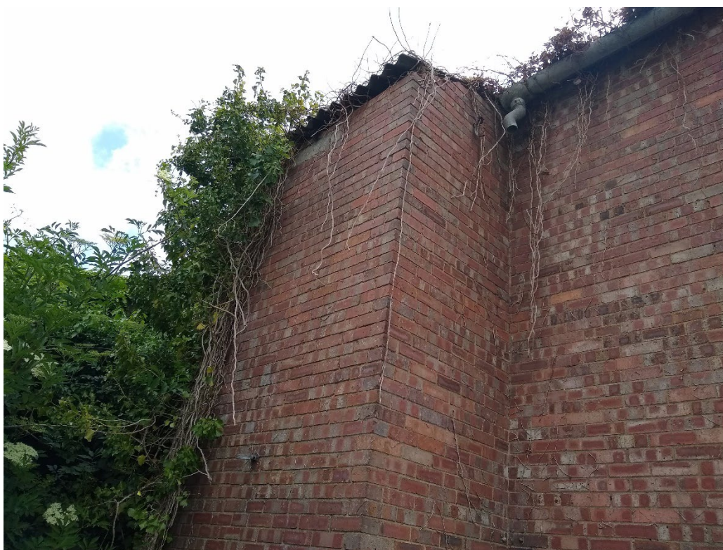
Photo 5 – Building B – north elevation.
