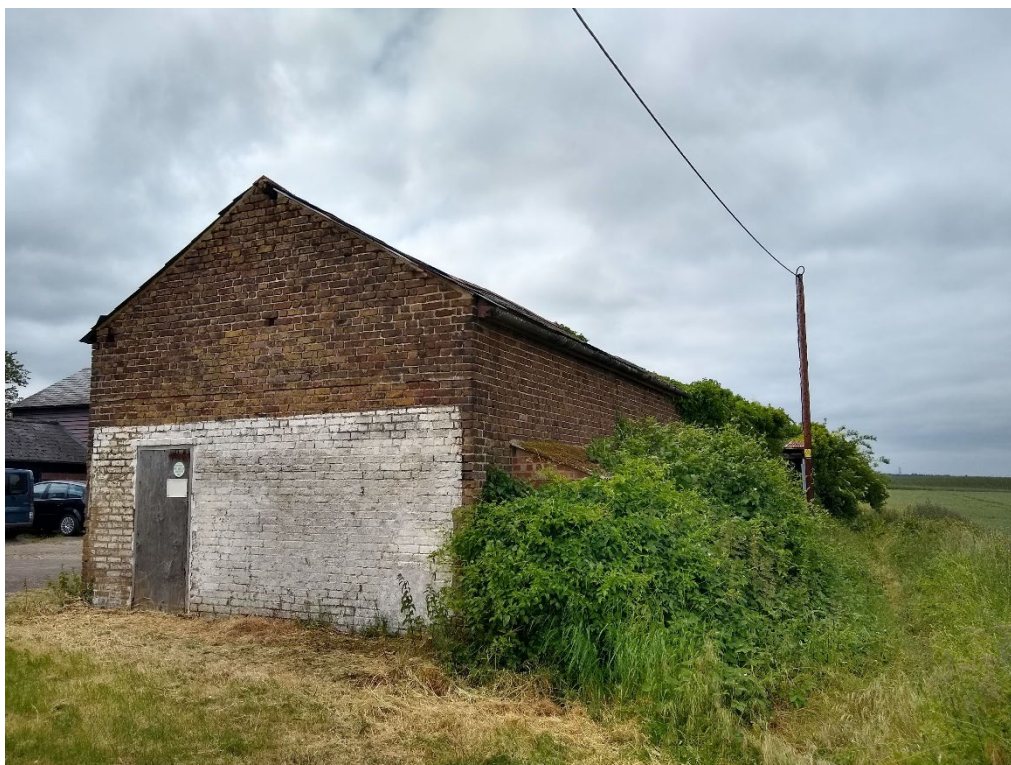
Photo 4 – Building A – east elevation.
