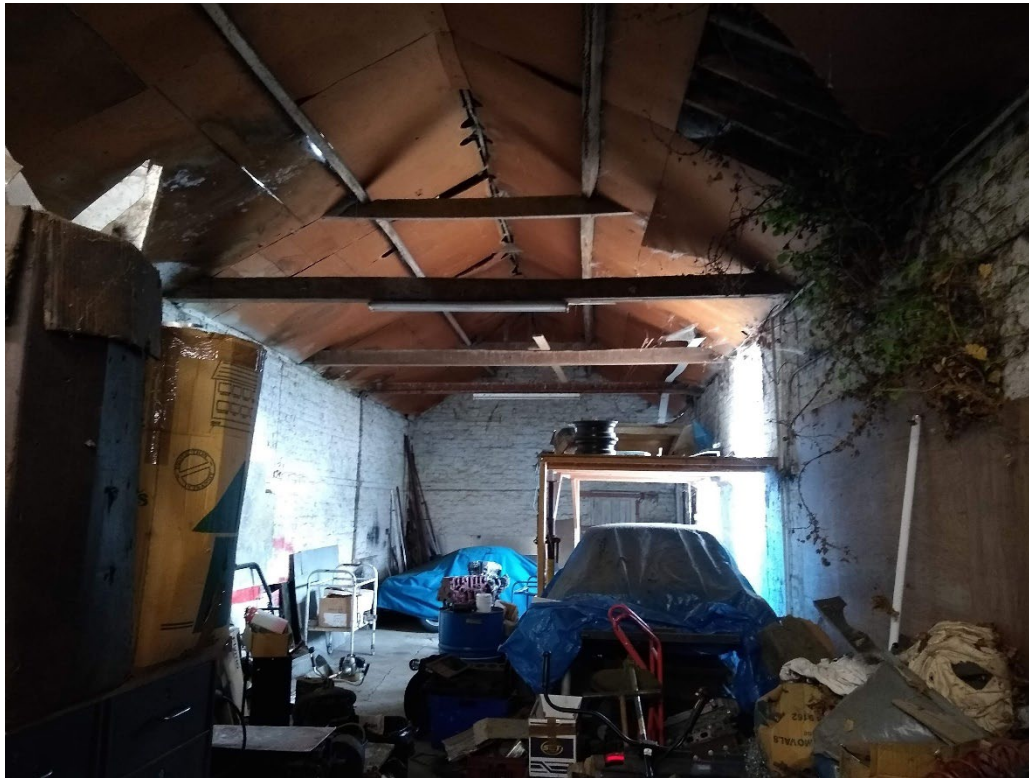
Photo 1 – Building A – internal.
