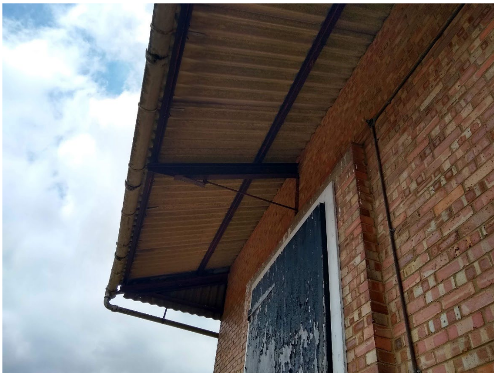
Photo 7 – Building B – canopy overhang.
