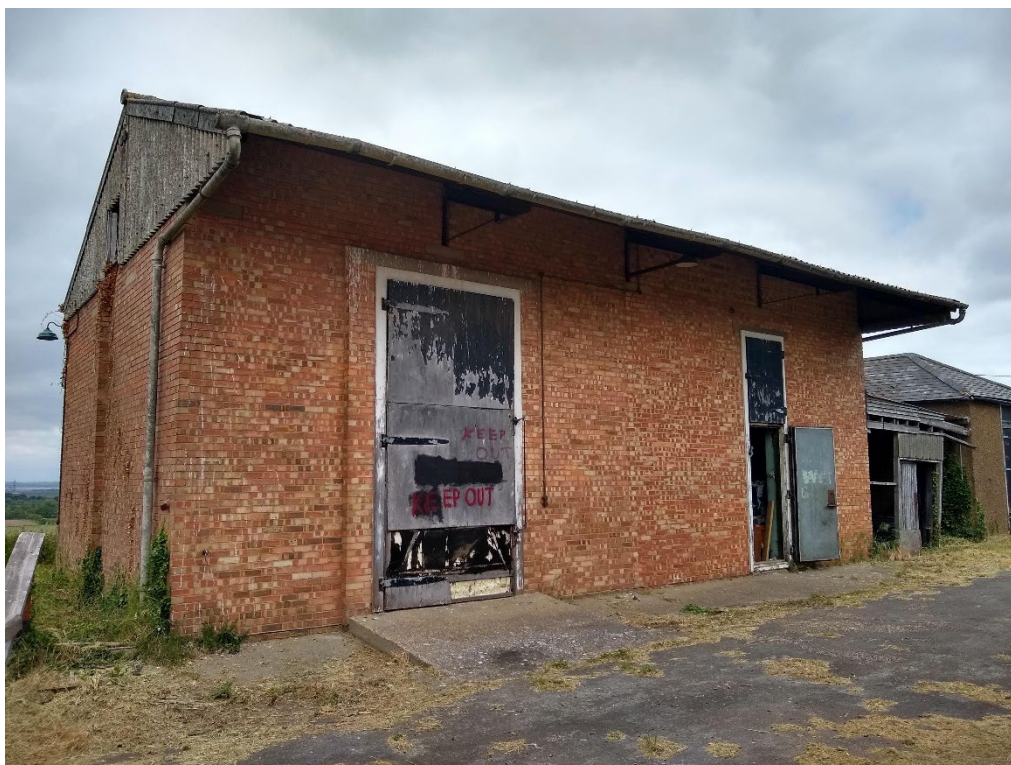
Photo 6 – Building B – south elevation.
