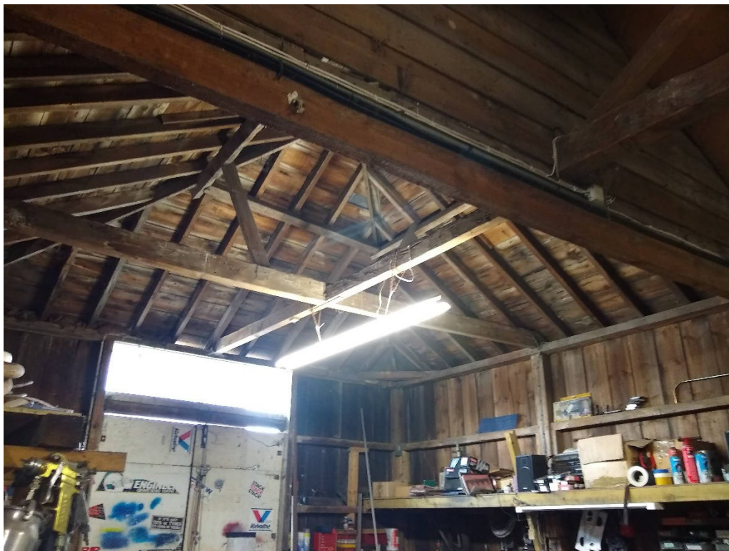
Photo 2 – Building A – internal.
