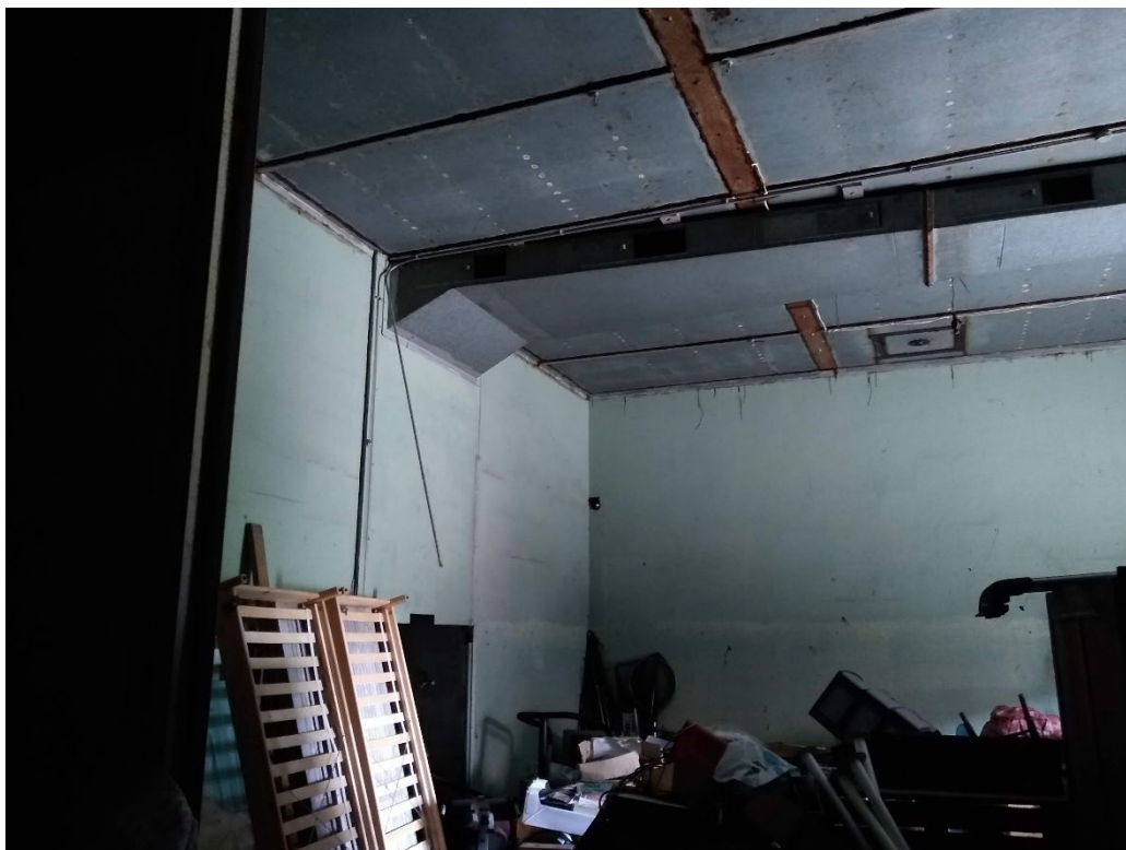
Photo 8 – Building B - internal.
