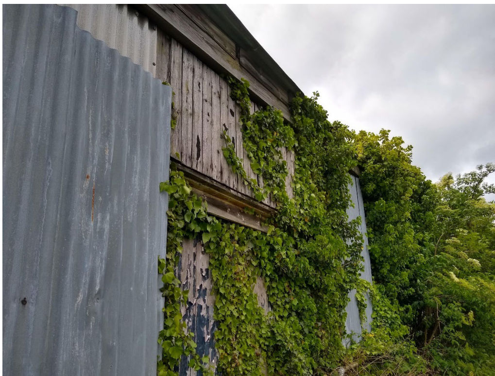
Photo 12 – Building C – north elevation.
