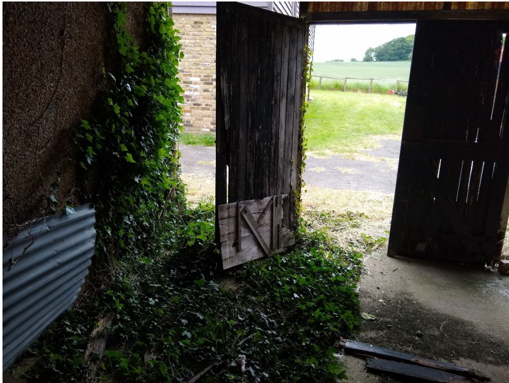
Photo 9 – Building C – internal view of south wall.
