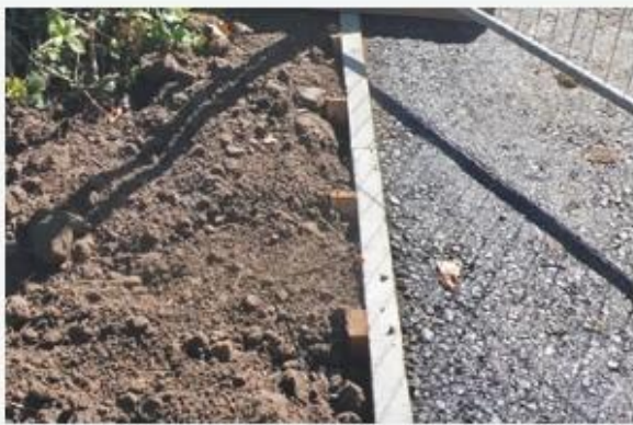
Small concrete kerbs pegged and set in concrete
