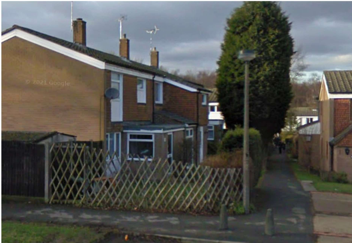
Front of No 15 Admers Wood
