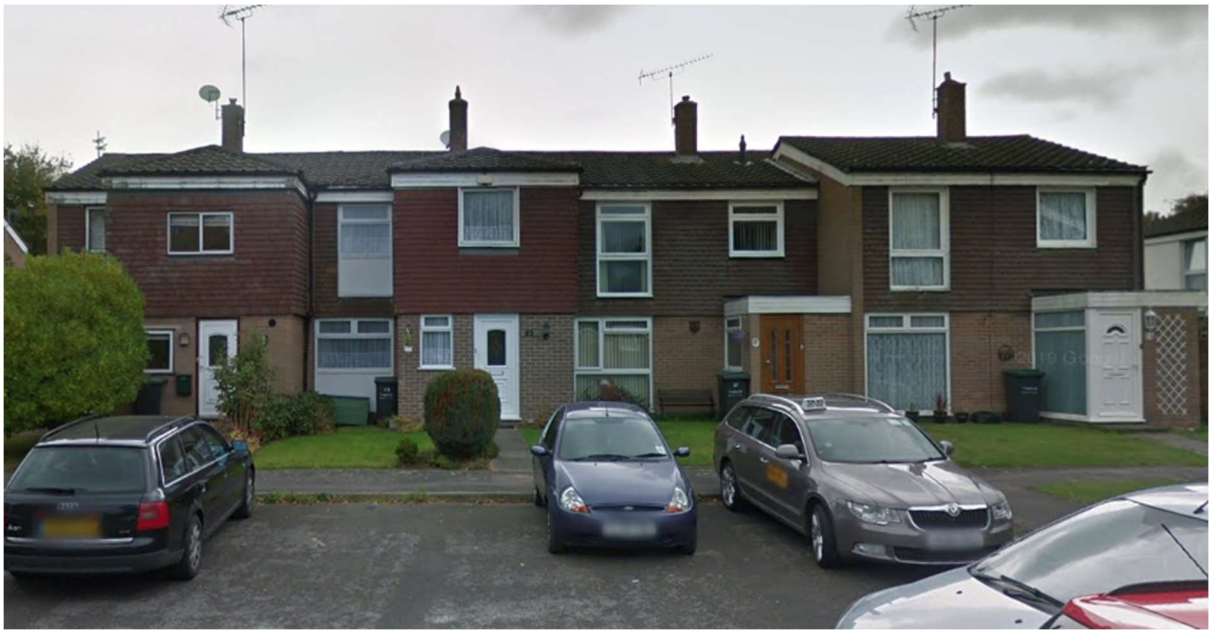
Front of No 15 & 16 Ferndown On a staggered terrace
