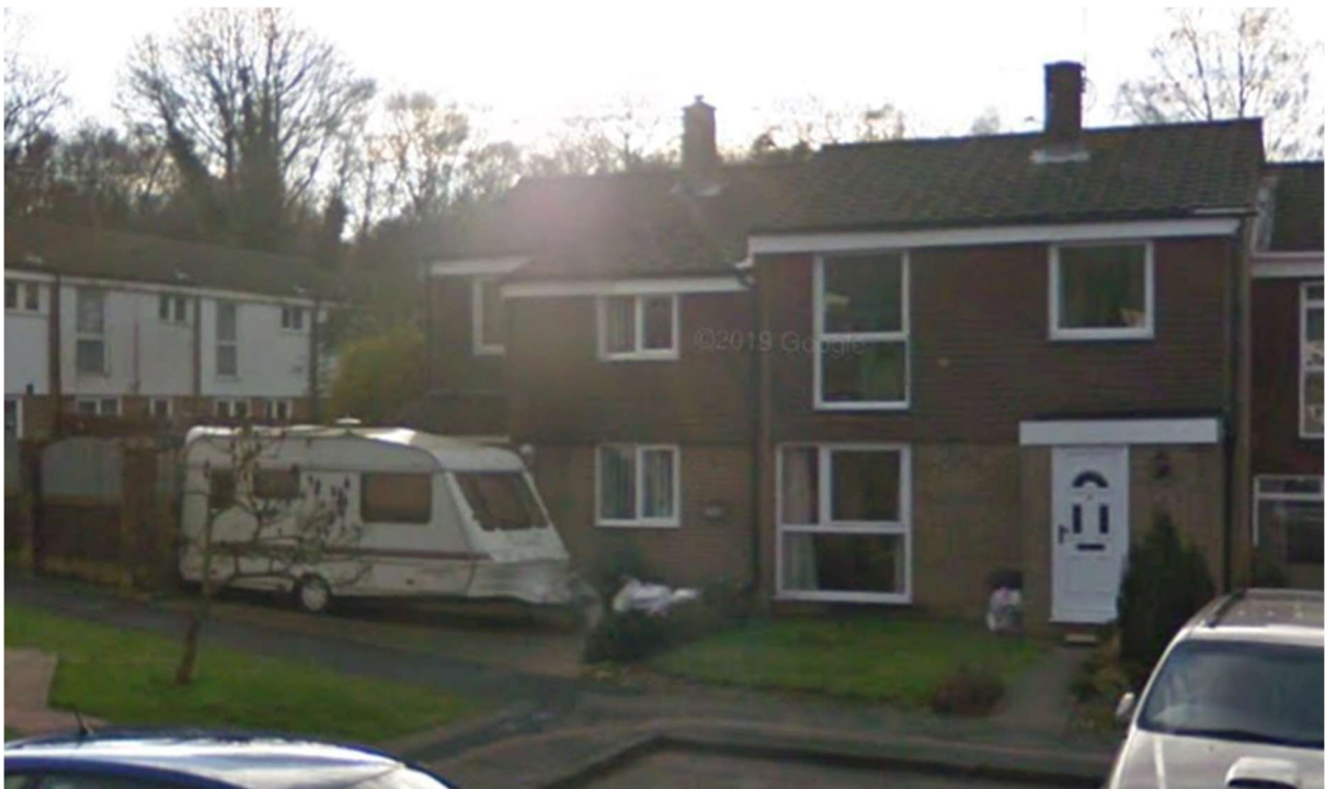
Front of No 7 Beech Mast, aligning to the front to the neighbour in a staggered terrace.
