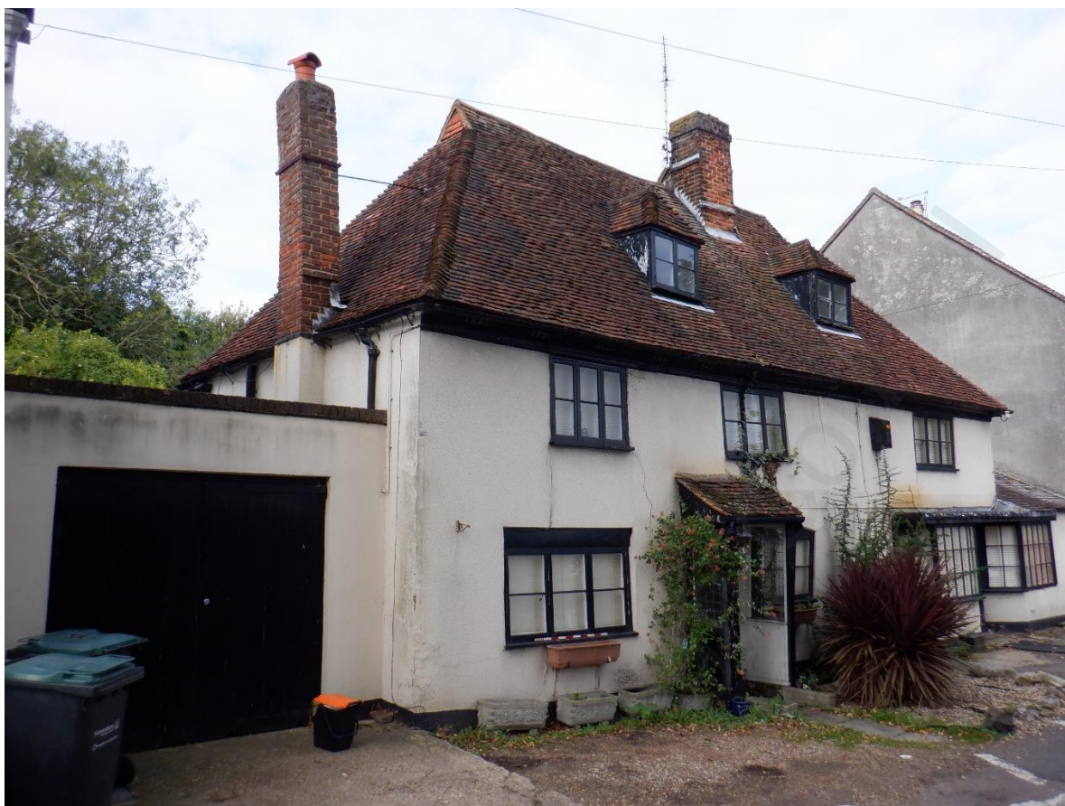
Plate 11. Frontage of the Old Post Office (looking NW)
