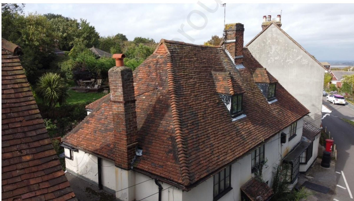
Plate 18. View of roof (looking NNW)
