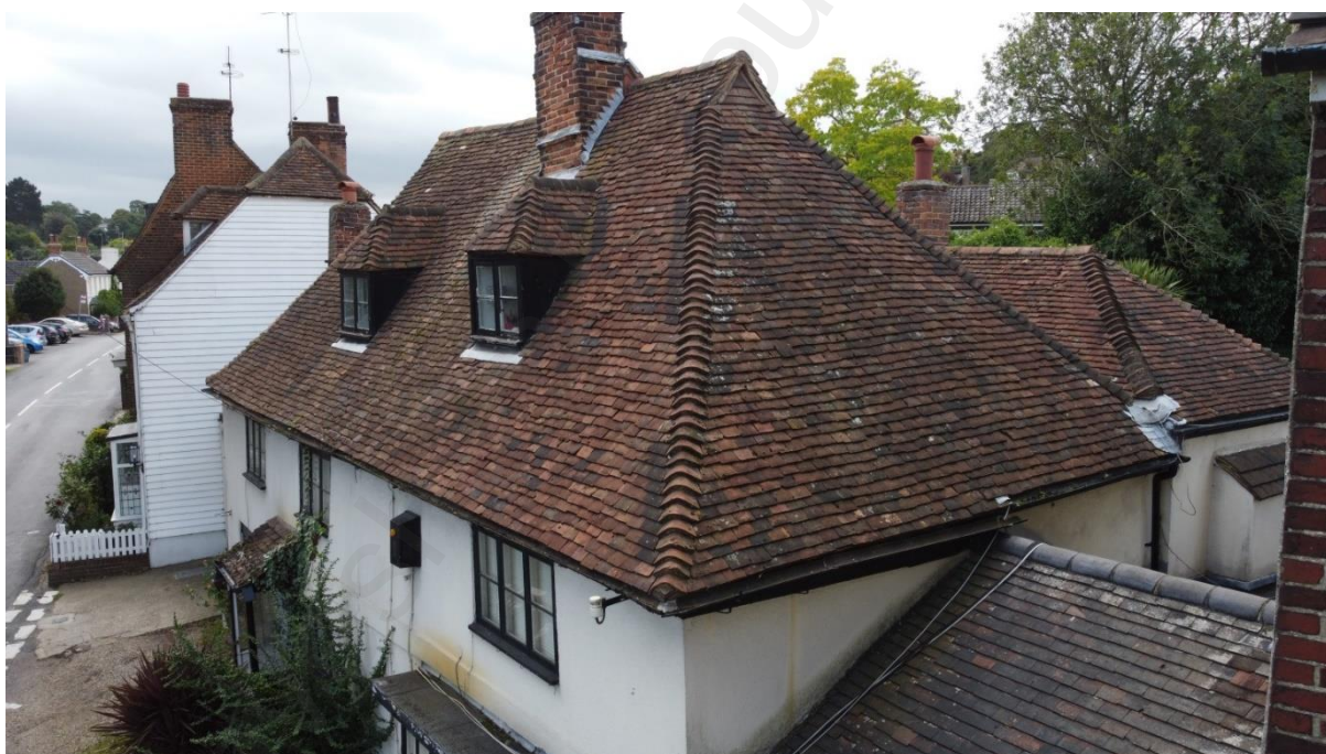
Plate 20. View of roof (looking South)
