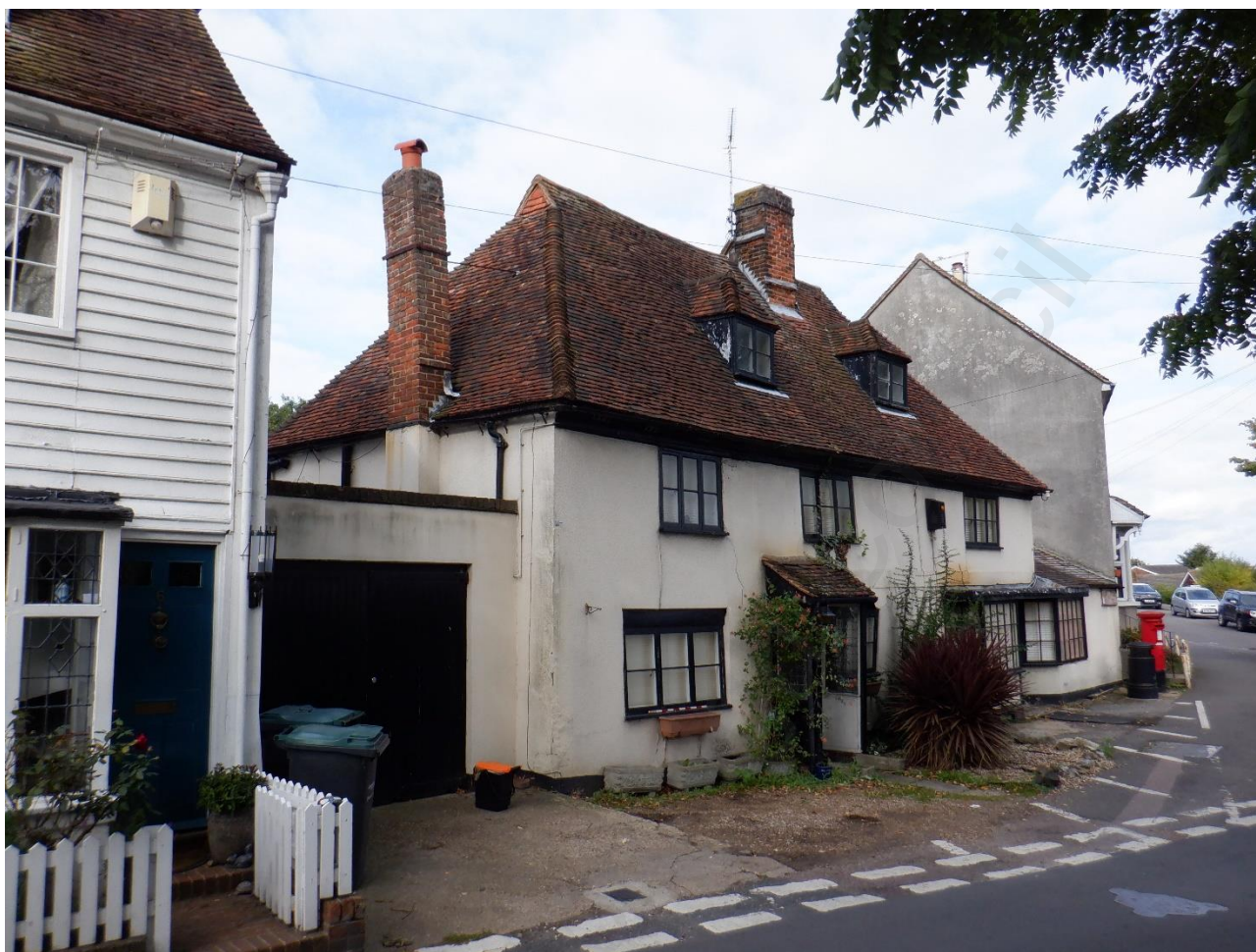
Plate 13. Frontage of the Old Post Office (looking NW)
