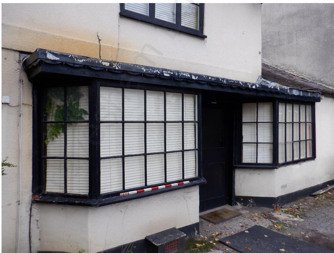
Plate 10. Frontage of the Old Post Office (detail looking NNW)
