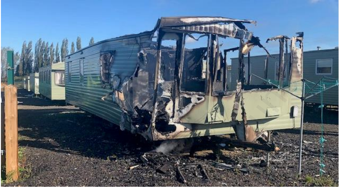
Figure 5 – Photo showing worker's accommodation that was damaged by a fire.
