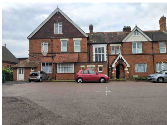
Existing 1950s extension in front of entrance to Theydon
