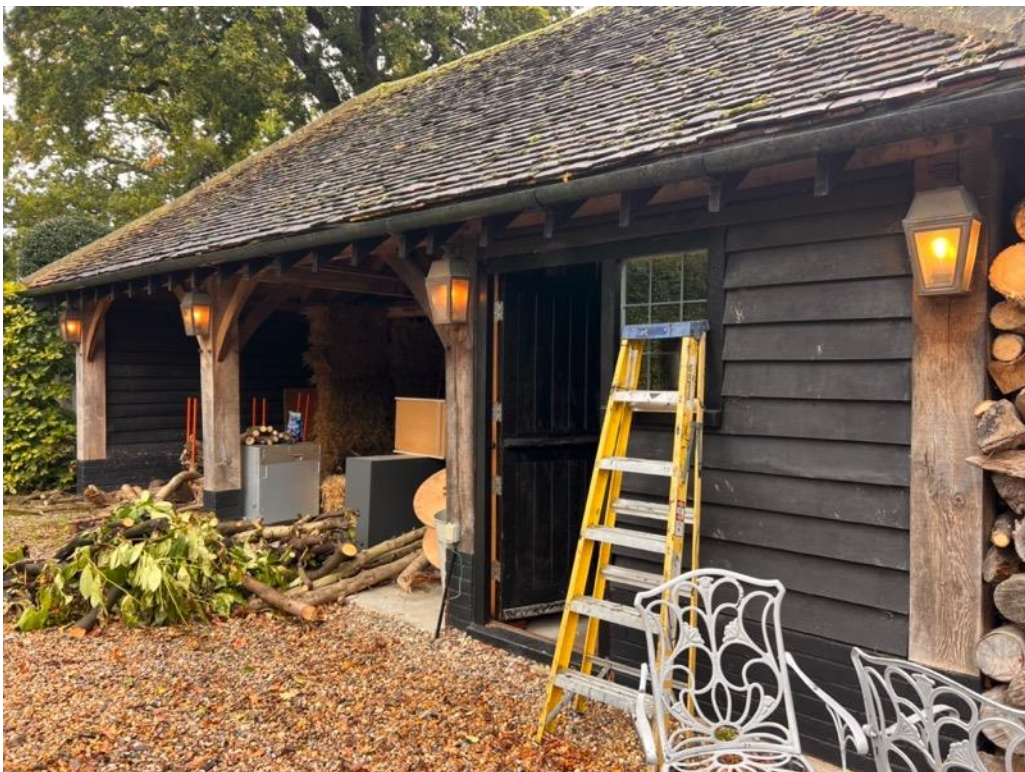
Views of the front elevation of the outbuilding from the driveway
