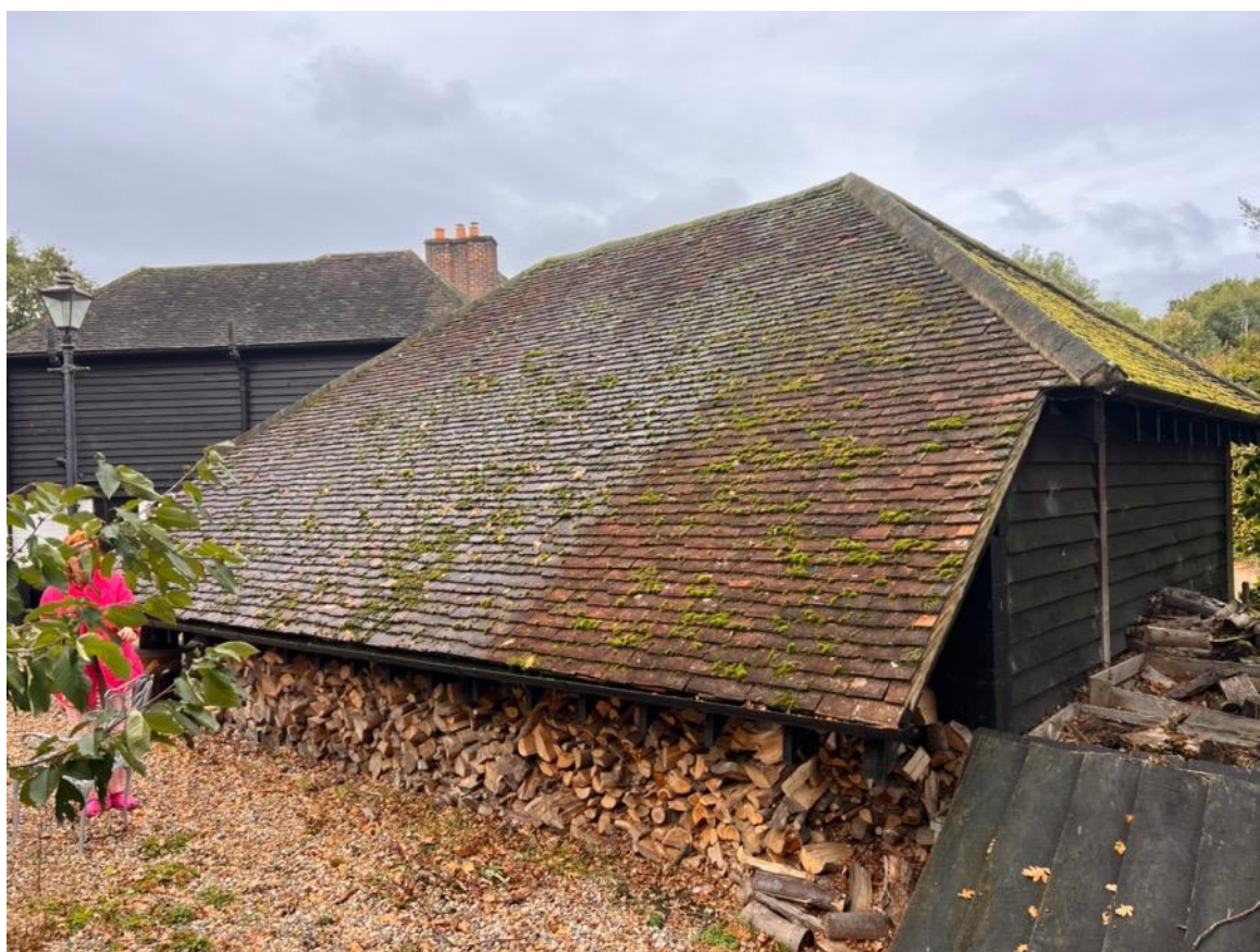
View of the rear and side (west) elevation of the outbuilding, with Wyebank visible in the background
