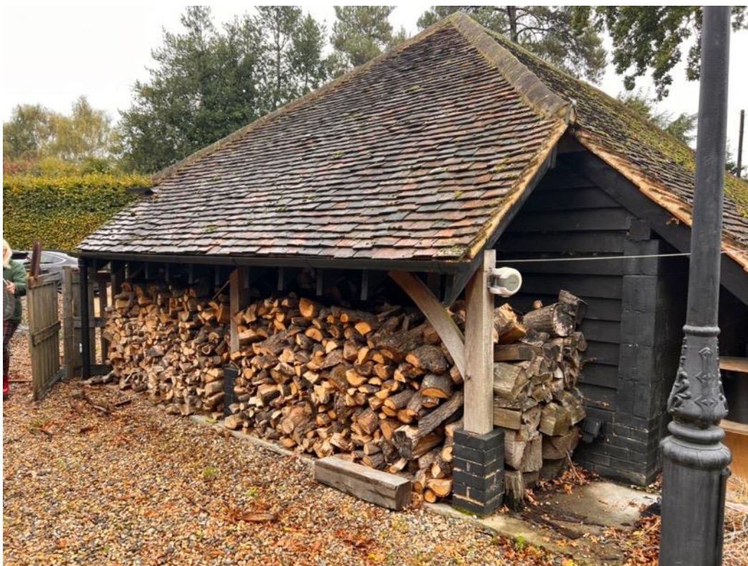
View of the side (east) elevation of the outbuilding, housing the covered log store
