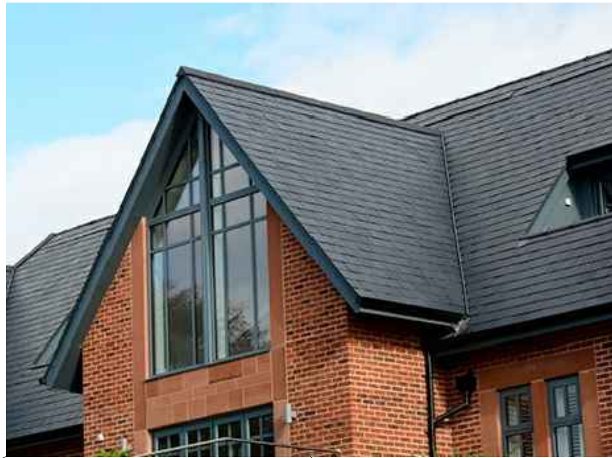
Natural slate roof
