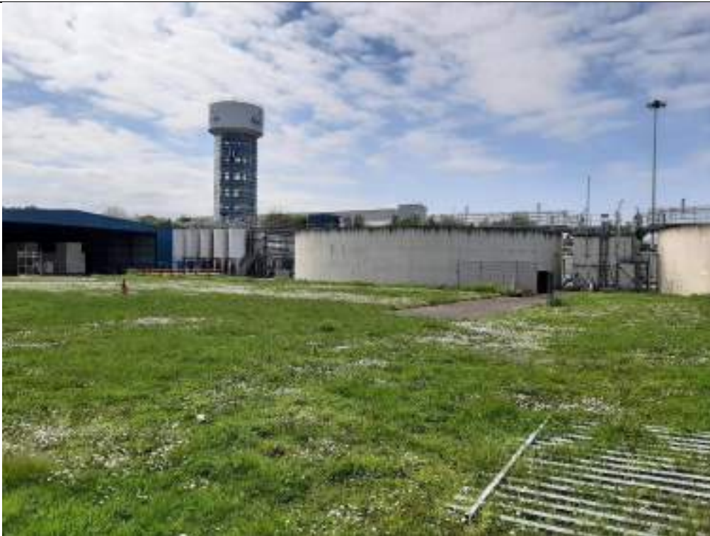
2. View SW – Water storage tanks on right (West)
