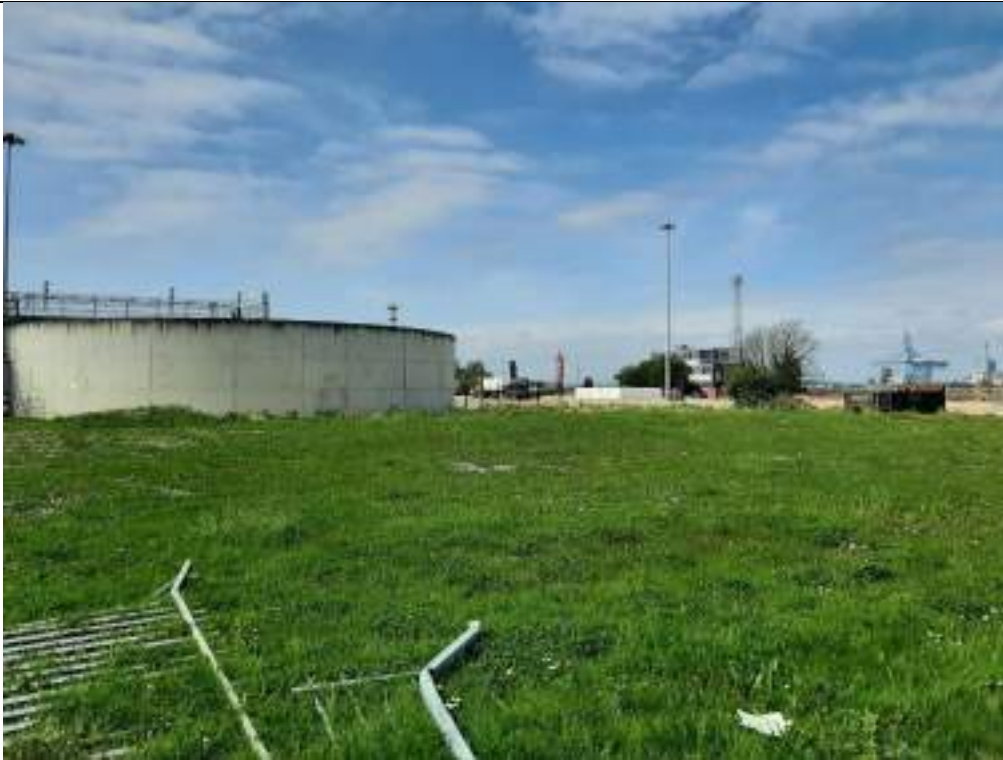
3. View NW, water storage tanks to left (West).
