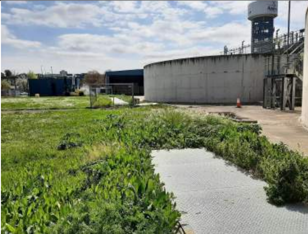
5. West side of site view to SW – service duct covers with water tanks to west.
