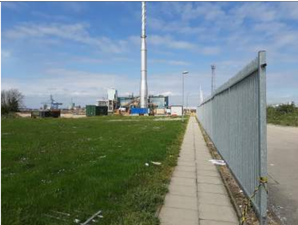
4. View North with Eastern boundary fence to right (East)
