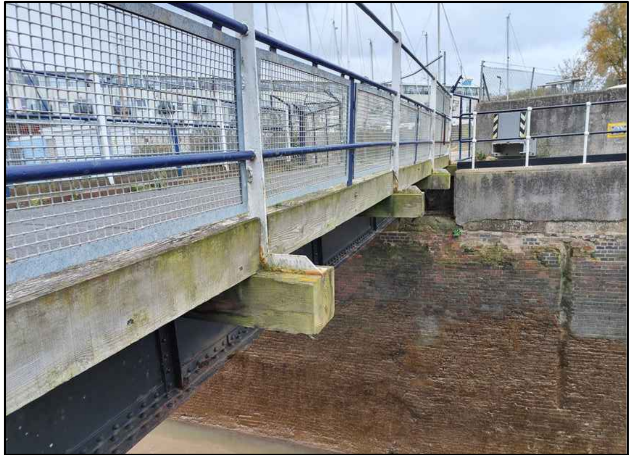
PHOTO 1 - ELEVATION TO SIDE OF EXISTING BRIDGE
