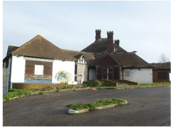
Photograph 2. Principal Building from the west.
