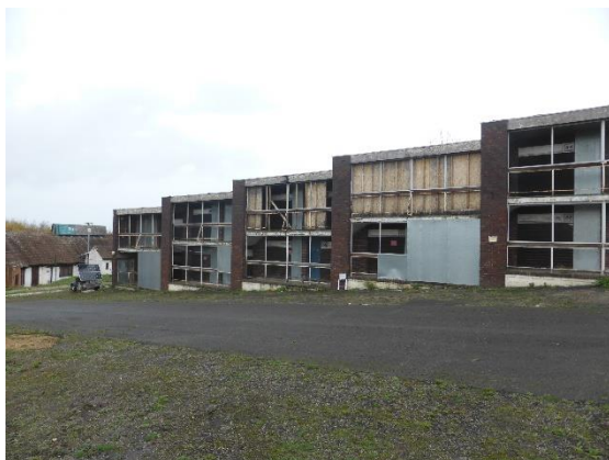
Photograph 7. Western Accommodation Block.
