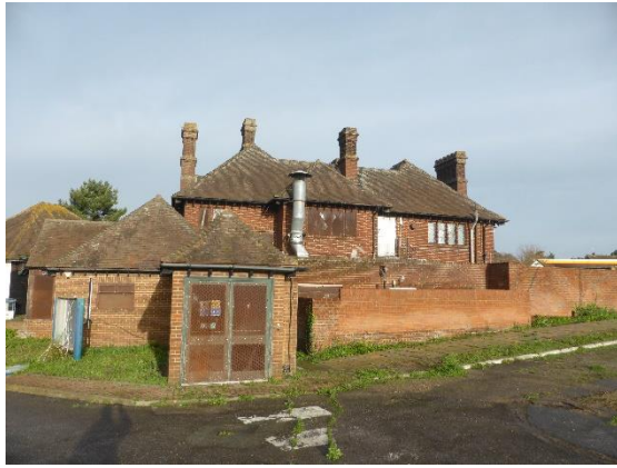
Photograph 1. Principal Building from the east.
