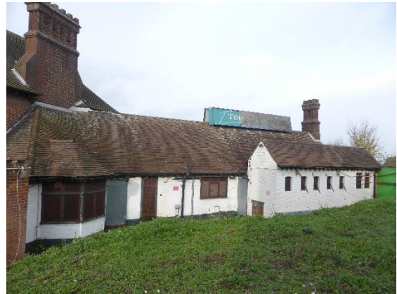
Photograph 4. Principal Building from the east.
