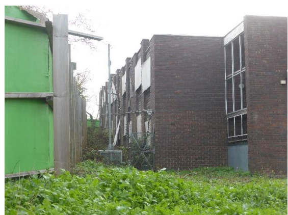
Photograph 6. Rear of the western Accommodation Block.
