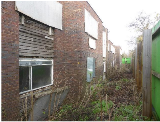
Photograph 9. Rear of Eastern Accommodation Block.
