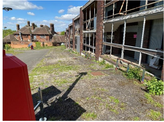
Photograph 20. Car park to Western Accommodation Block.
