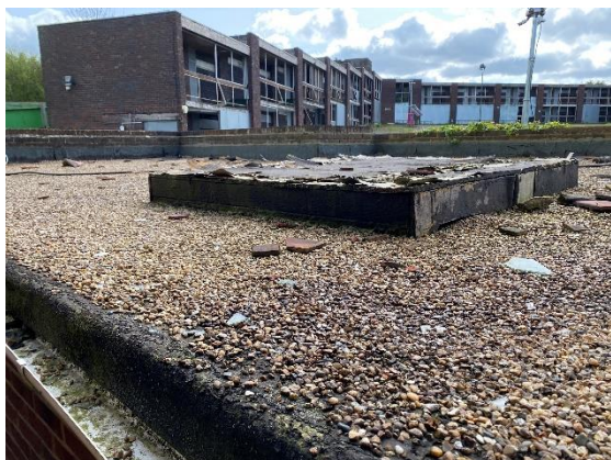
Photograph 7. Flat roof over extension to Principal Building.
