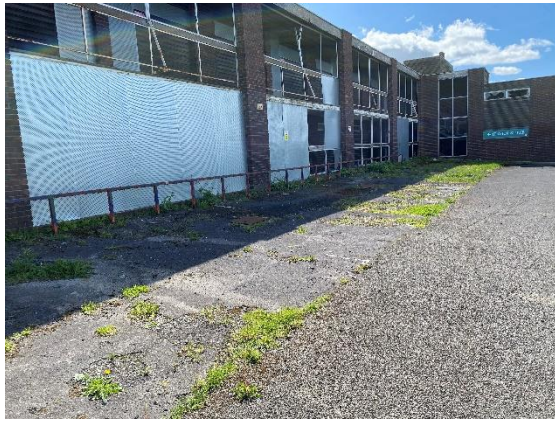
Photograph 19. Car park to Eastern Accommodation Block
