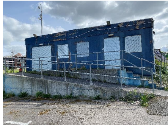
Photograph 18. Temporary Building for security office.
