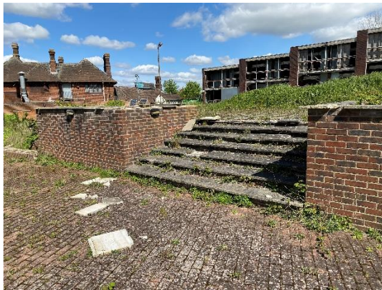
Photograph 21. Steps and paving to north of Function Room.
