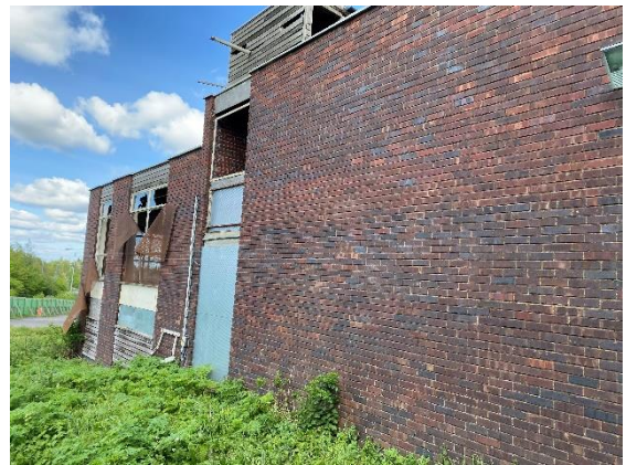
Photograph 12. Rear of Eastern Accommodation Block.
