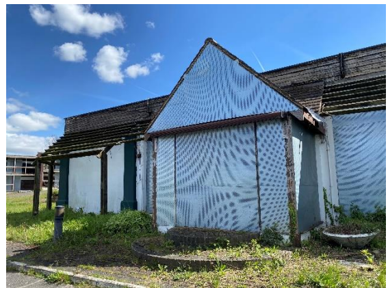
Photograph 16. Function Room Entrance.
