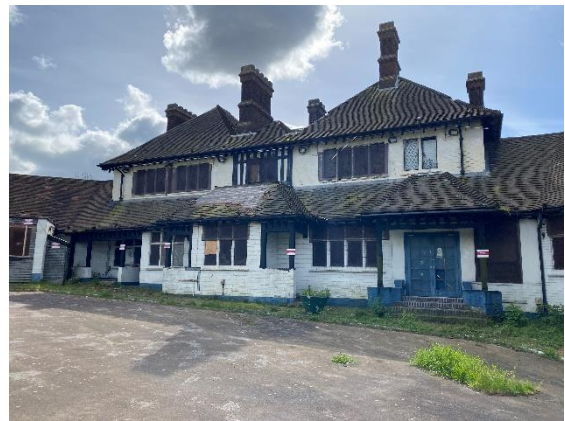
Photograph 4. Principal Building from the north.
