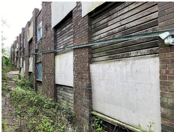
Photograph 11. Rear of Western Accommodation Block
