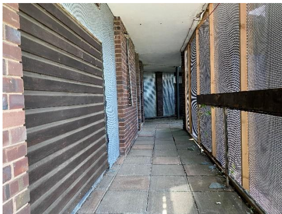
Photograph 13. Walkway to Accommodation Block.
