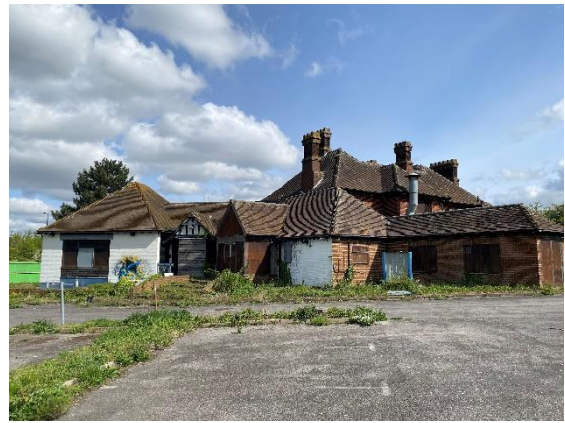
Photograph 2. Principal Building from the south.
