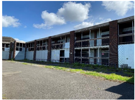
Photograph 10. Front of Eastern Accommodation Block
