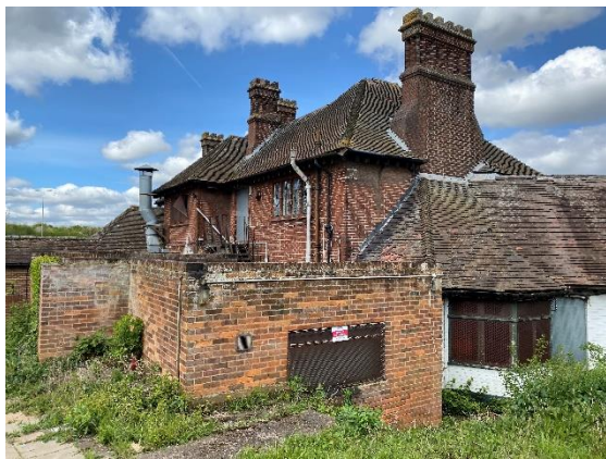
Photograph 5. Principal Building from the north.
