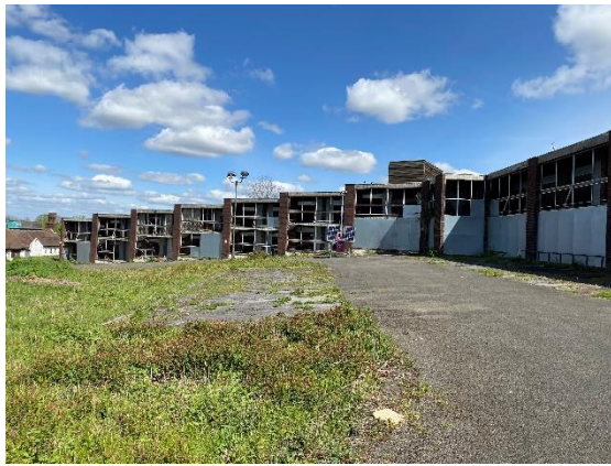
Photograph 9. Front of Western Accommodation Block.
