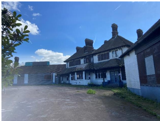
Photograph 3. Principal Building from the north.
