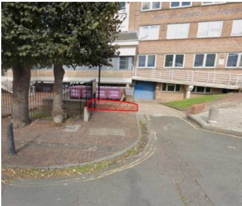
Figure 2: Bull nose to wall to be demolished as part of the works
