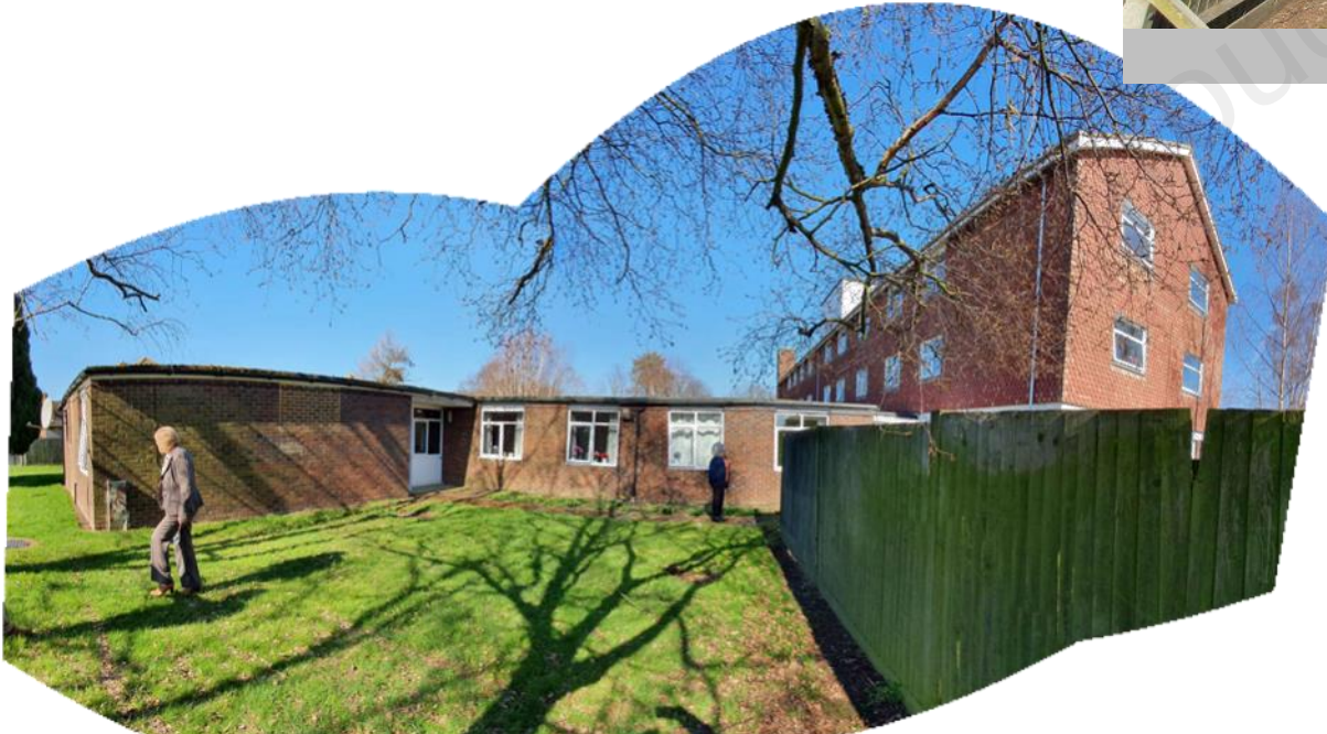
Fig 8—Hever Court Main single storey extension
