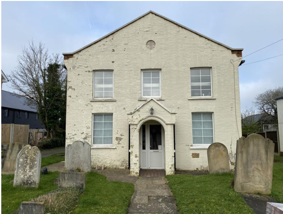
FRONT (EAST) ELEVATION PRIOR TO REMOVAL OF PAINT FINISHES
