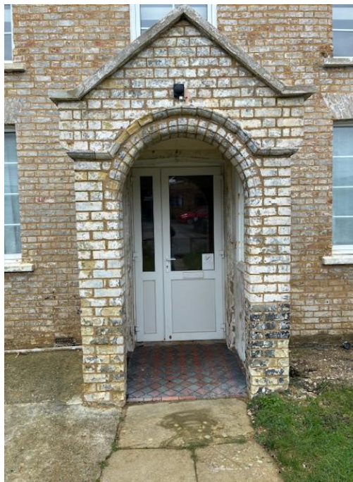
ENTRANCE PORCH AFTER REMOVAL OF PAINT FINISHES
