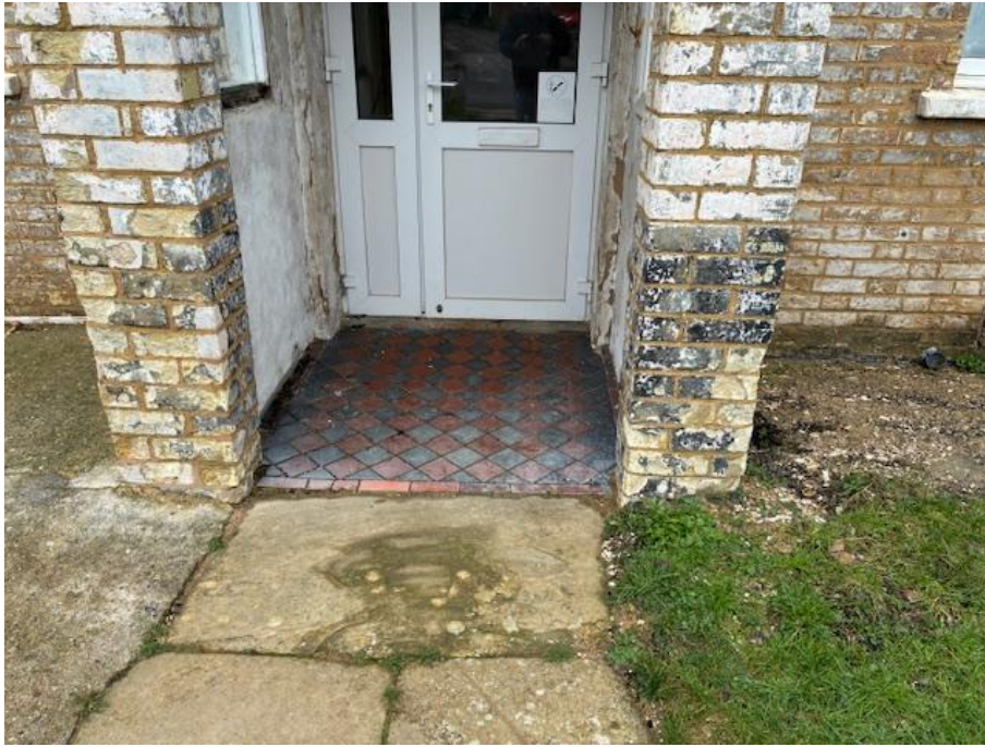
ENTRANCE PORCH LOWER FACADE AFTER REMOVAL OF PAINT FINISHES
