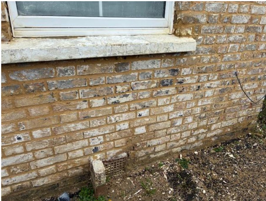
MAIN LOWER FACADE AFTER REMOVAL OF PAINT FINISHES
