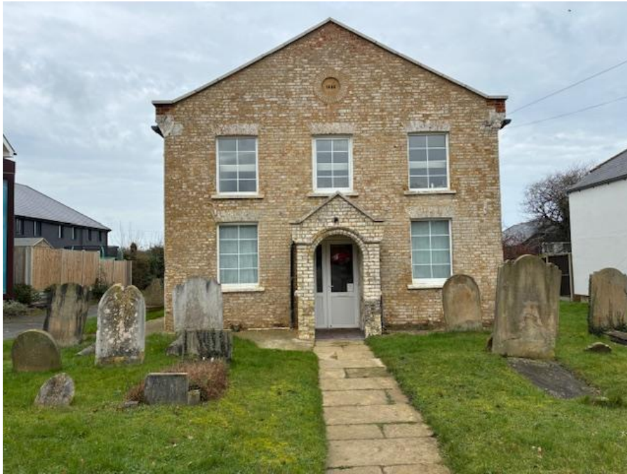
FRONT (EAST) ELEVATION AFTER REMOVAL OF PAINT FINISHES
