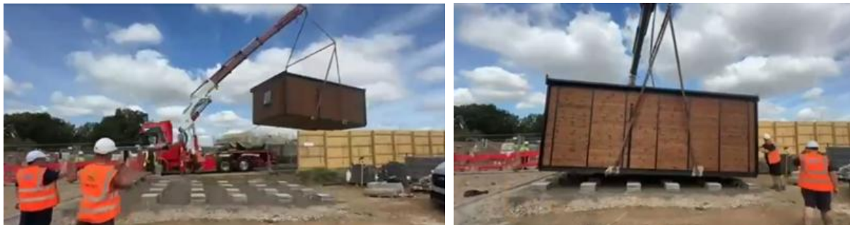
Figure 3: Lifting capability of the proposed mobile home, using a crane to remove it from the land.
