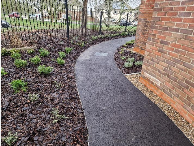
Figure 1. Footpath between T01 and T02 and the new building.
