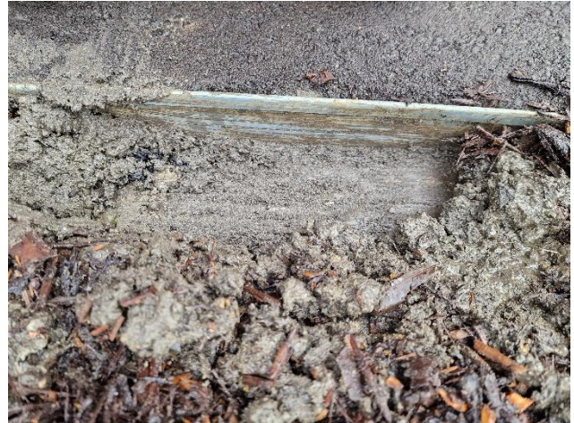
Figure 2. Footpath concrete sub-base or haunching.
