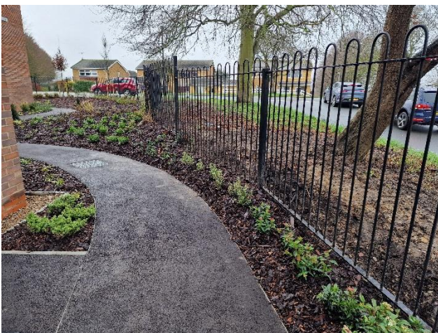
Figure 3. New fence post adjacent to T02 with evidence of root severance.
