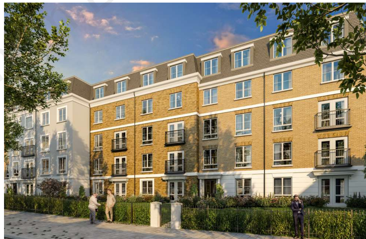
FIGURE 12: WINDMILL STREET FRONTAGE - LOOKING SOUTH WEST
