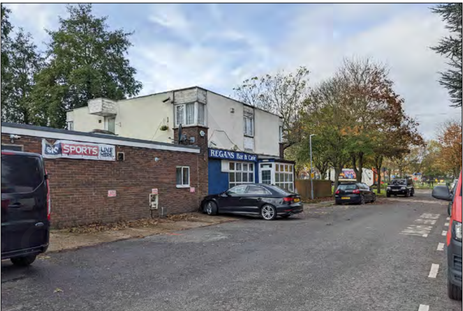
Photo 3) Cafe building between leisure centre buildings and car park viewed from the north.
