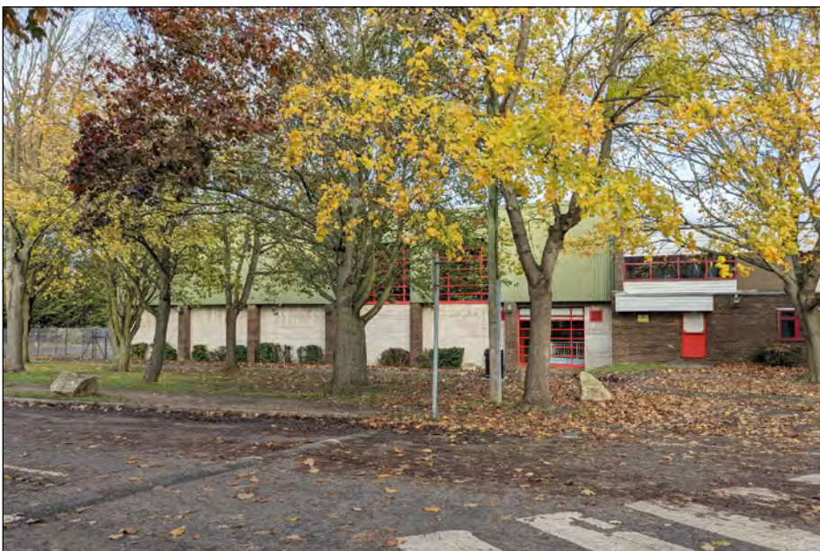
Photo 2) Western end of the present leisure centre buildings viewed from south side.
