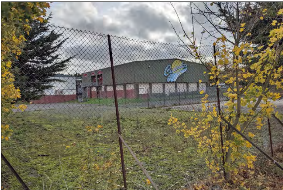
Photo 4) Western side of the present leisure centre buildings with tennis court area viewed from west.
