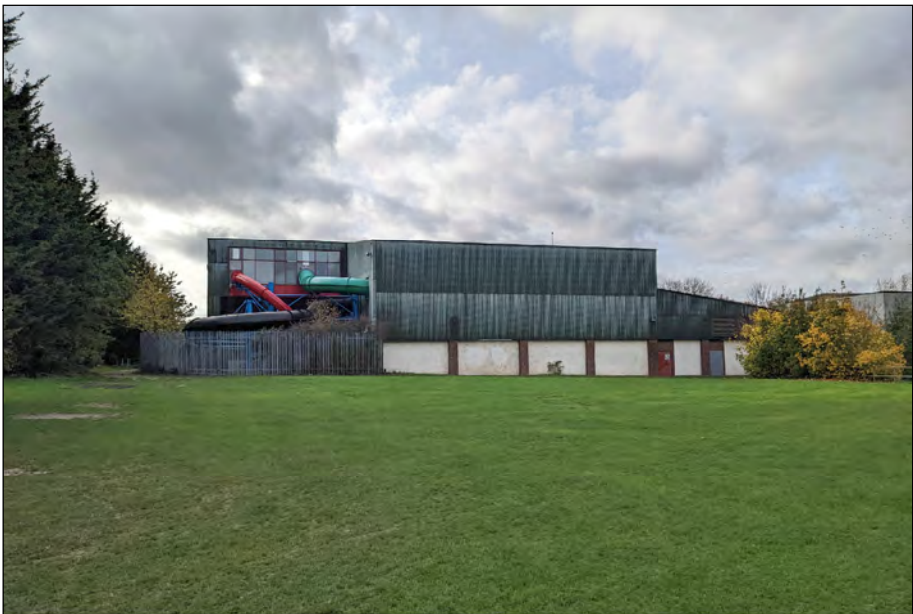
Photo 6) Leisure centre buildings viewed from the north with adjacent lawn in northern area of the site.
