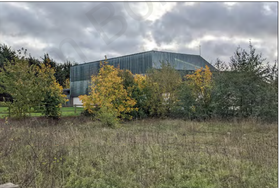
Photo 5) Northern side of leisure centre buildings viewed from north-west.
