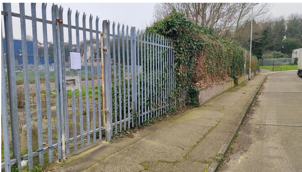
The buildings to be demolished are visible in this view.
