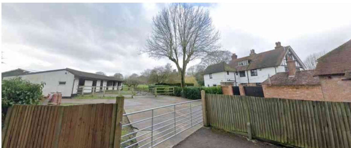
Plate 1 – Woodlands Farmhouse, ancillary buildings, including a Stable looking south-west across the PDA.
