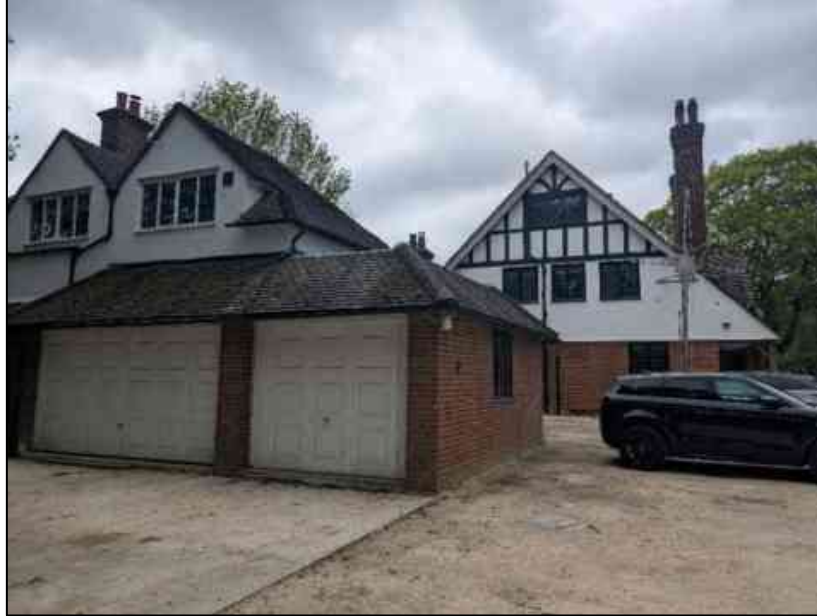
Plate 12. Northern elevation of Woodlands Farmhouse
