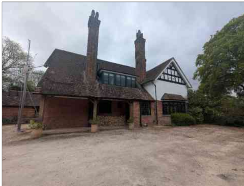
Plate 9. Western elevation of Woodlands Farmhouse
