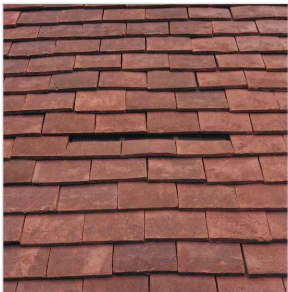
Keymer Clay In-line roof vent Installed
