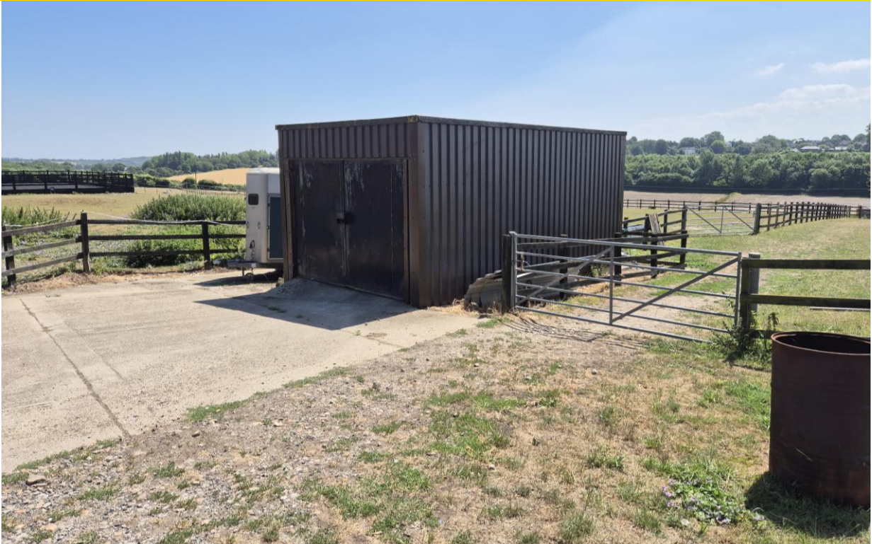
The existing storage container to be relocated.
