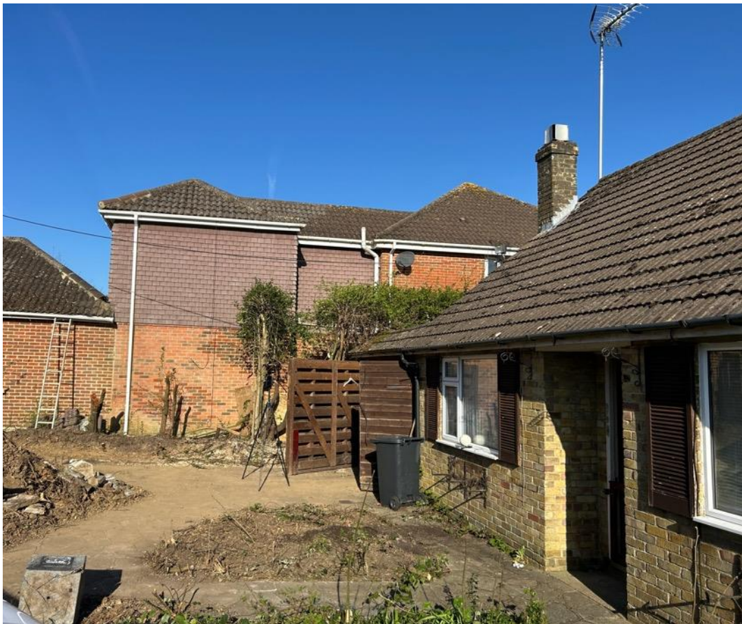
View towards adjacent two storey house, Three Jays, to the west.
