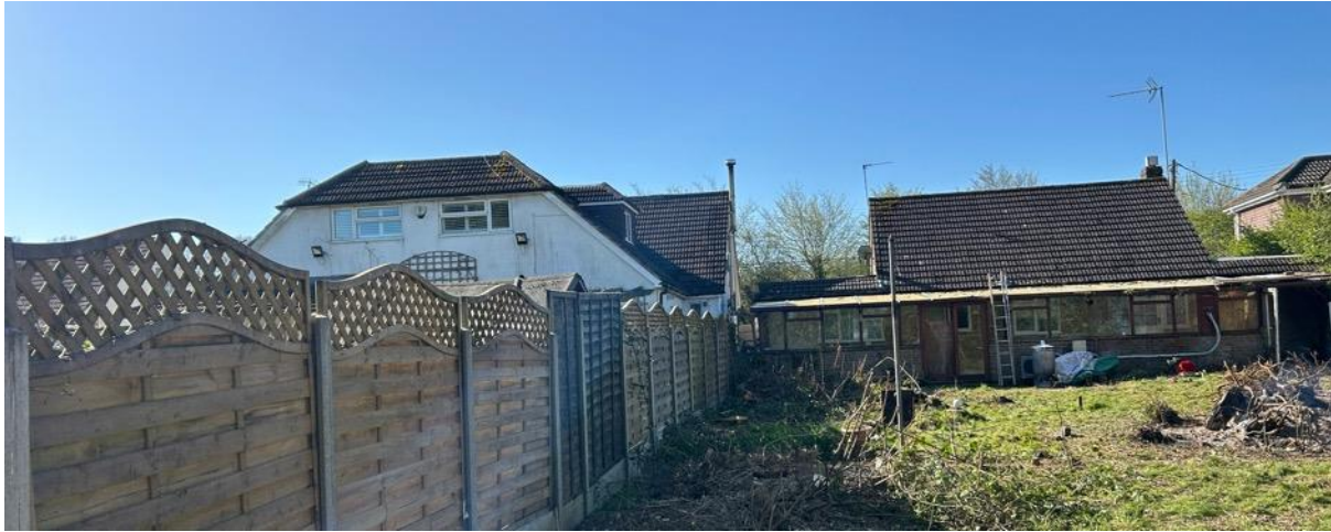
Rear of existing bungalow indicating two storey element to the rear of Brackenwood.
