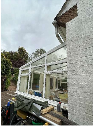
Conservatory from West side
