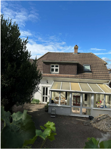
Conservatory Rear of No 125, showing screening trees to left hand side
