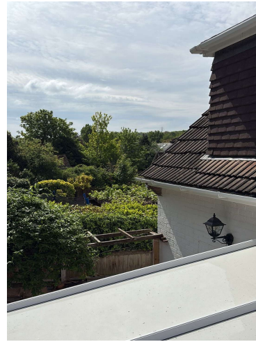
View from above existing conservatory looking South toward No 127
