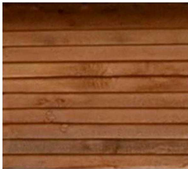
Horizontal Timber Featheredged Boarding
