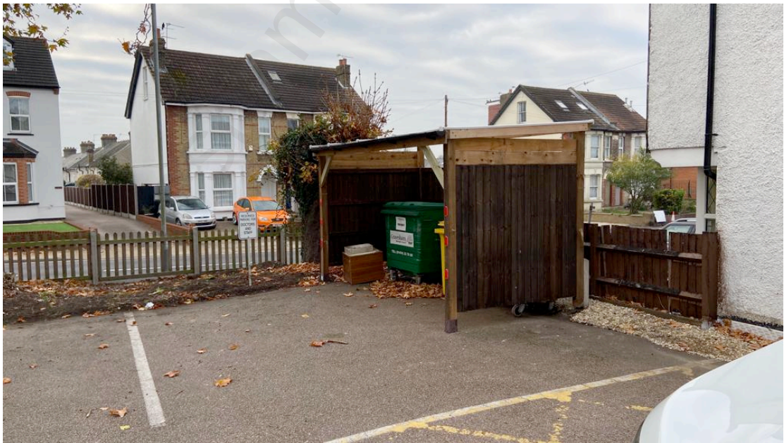
Fig 1 Existing site view taken car park facing Old Road West
