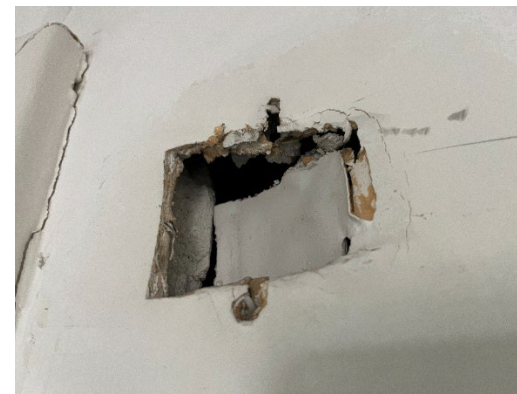
Third Floor details – two rooms with the same window configuration, area of fitting removed to show modern wall construction
