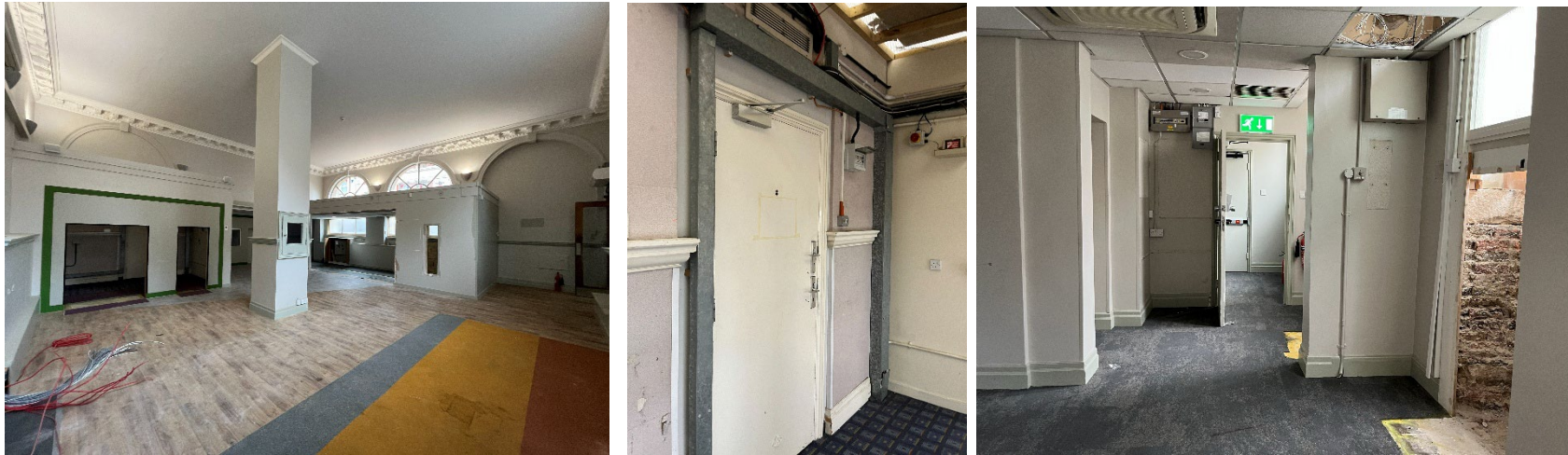
Ground Floor Banking Hall, and rear subdivided areas with inserted services in many locations
