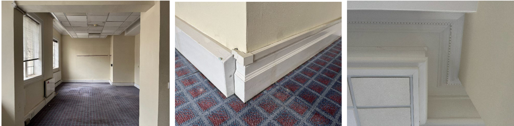
Typical First Floor condition – modern fit out but with some surviving cornice in front rooms
