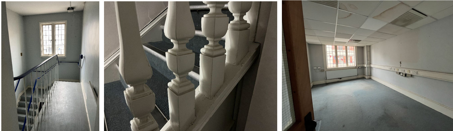
First floor details - 1930s rear staircase, original central staircase, typical room
