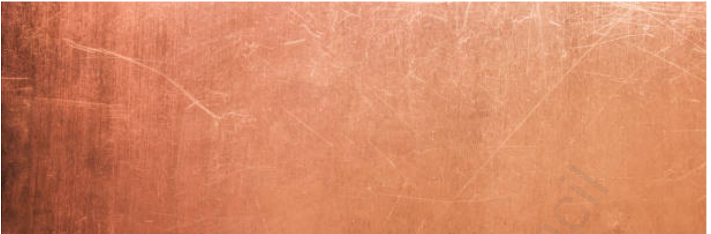
Copper band to rear extension fascia.
