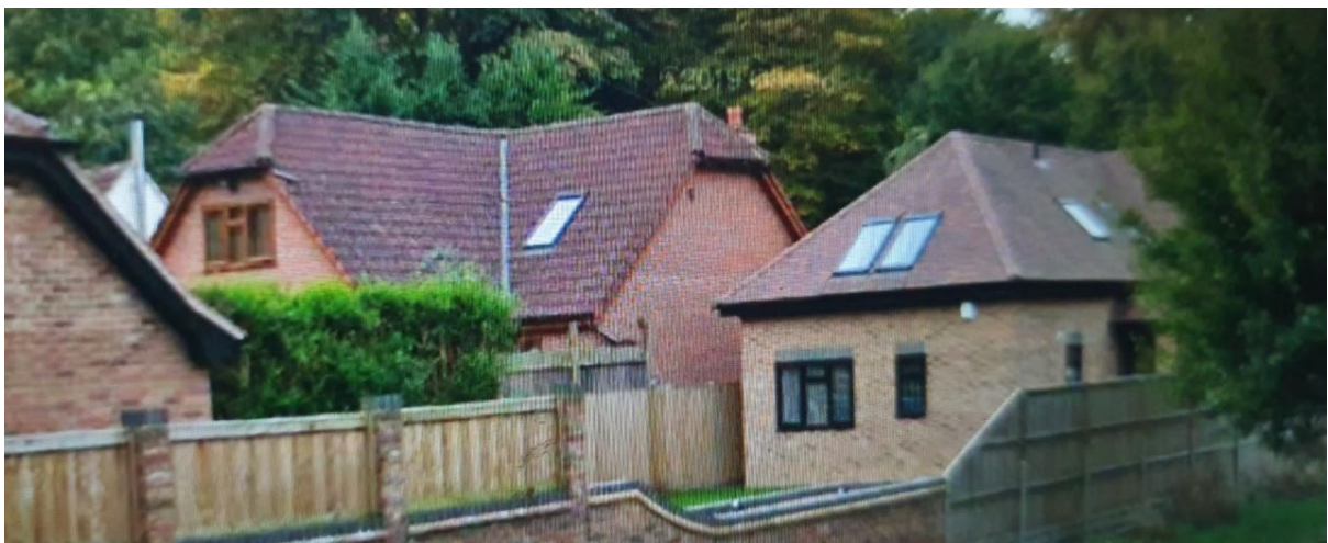
Modern built mixed material and sized properties 500m from "The Den" Plot
