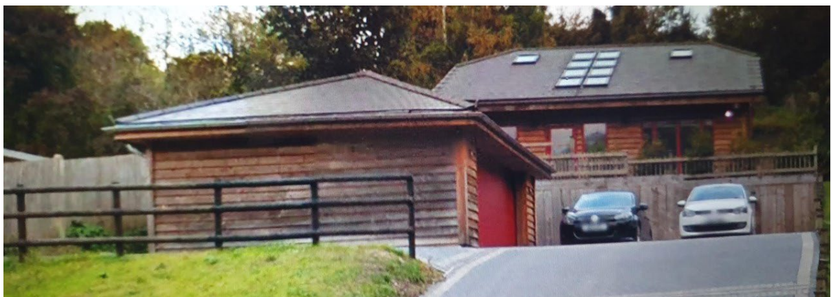
Modern mixed material – timber cladding and slate effect roof tiles
