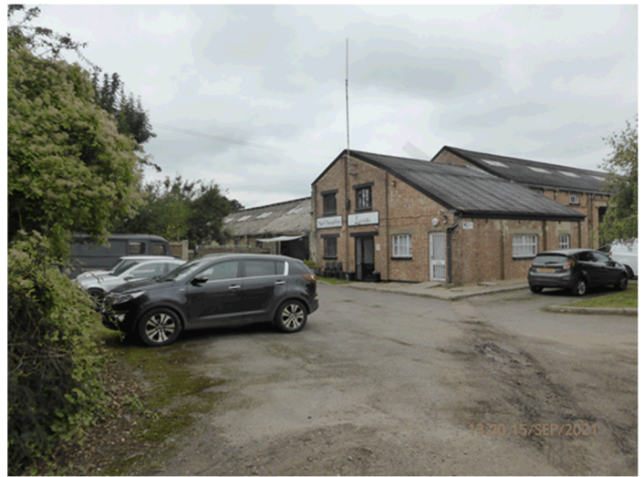
Some buildings on the Lomer Farm Estate
