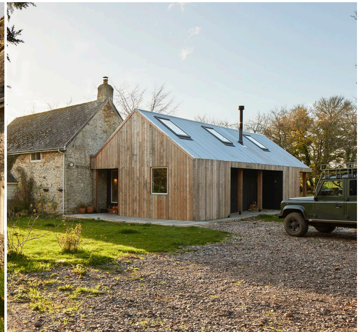
Precedent - Contemporary materials and flush rooflights
