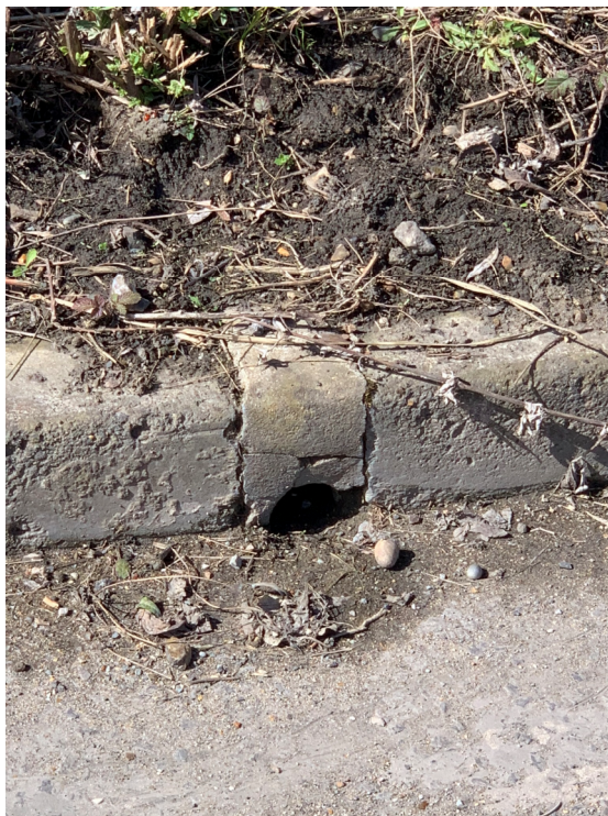
Figure 1: Tilbury existing road drainage.
