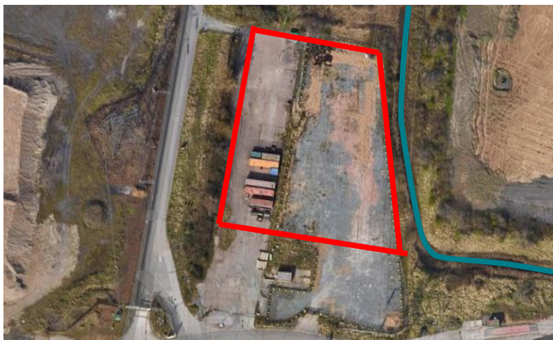
Figure 3: Aerial image of proposed Tilbury site area (ditch in blue).
