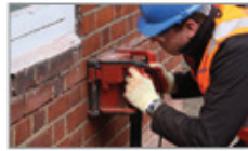
1. Rake out or cut slots into the horizontal mortar beds, a minimum of 20" either side of the crack.
