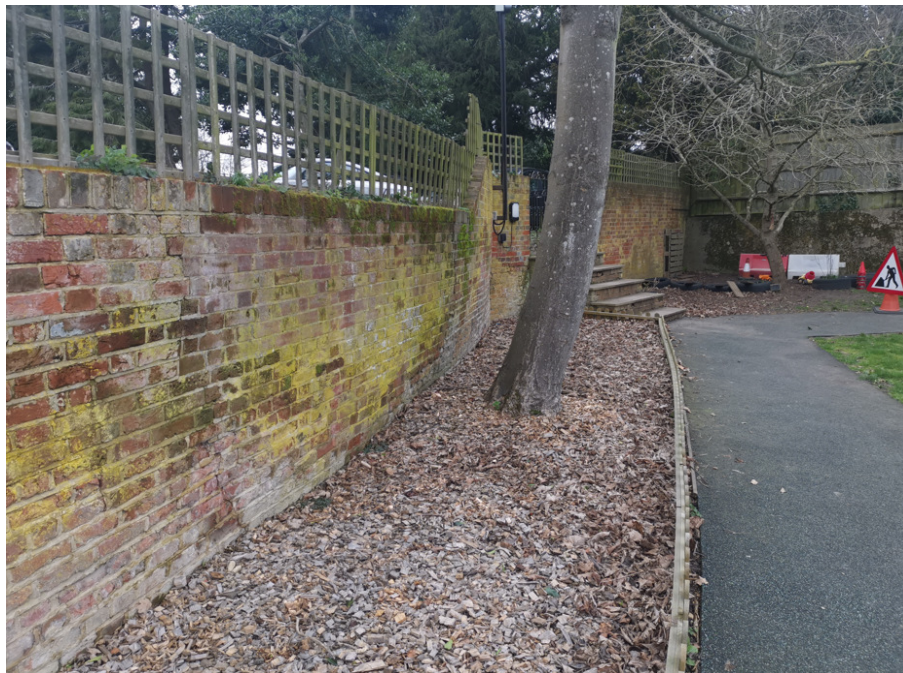
P005 – retaining wall looking north
