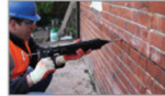
5. Insert a further bead of HeliBond over the exposed HeliBar, finishing 1/2" from the face, and 'iron' into the slot using the brick jointer.
