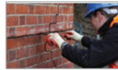
4. Using the brick jointer, or similar, push one HeliBar into the grout to obtain good coverage.
