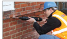
3. Using the HeliFix Pointing Gun Kit, inject a bead of HeliBond along the back of the slot.
