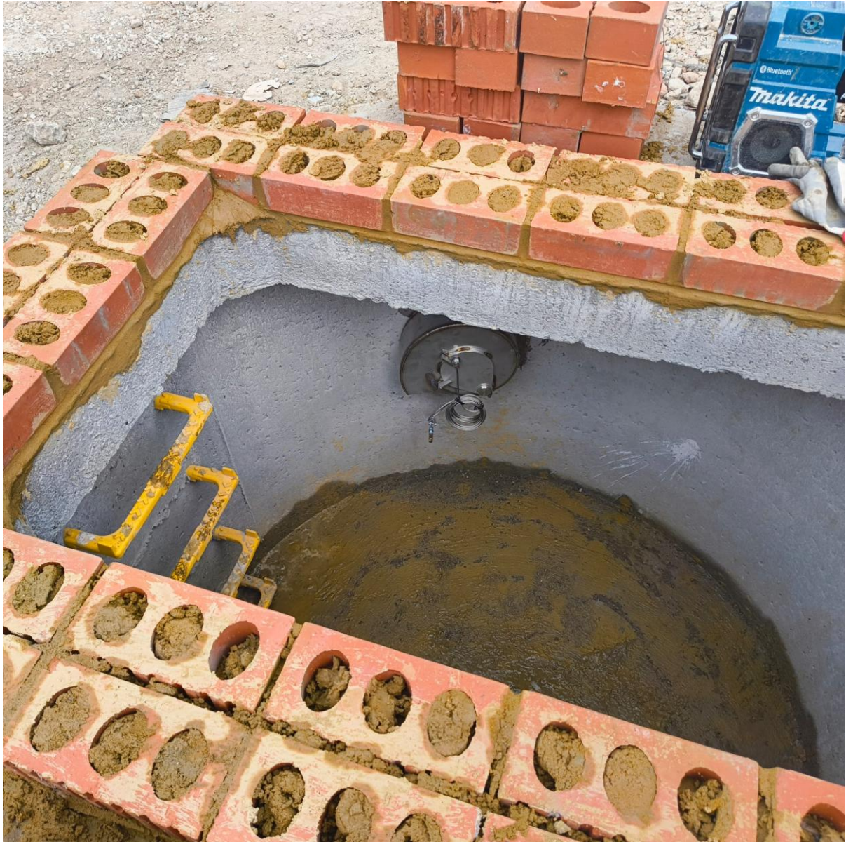
Hydrobrake installation
