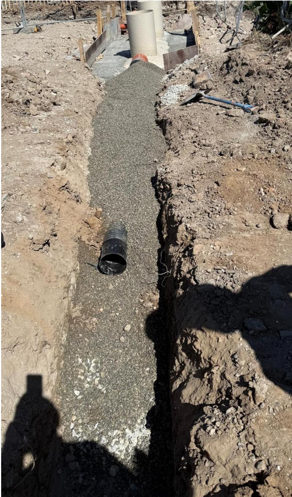
Drain run from Interceptor
