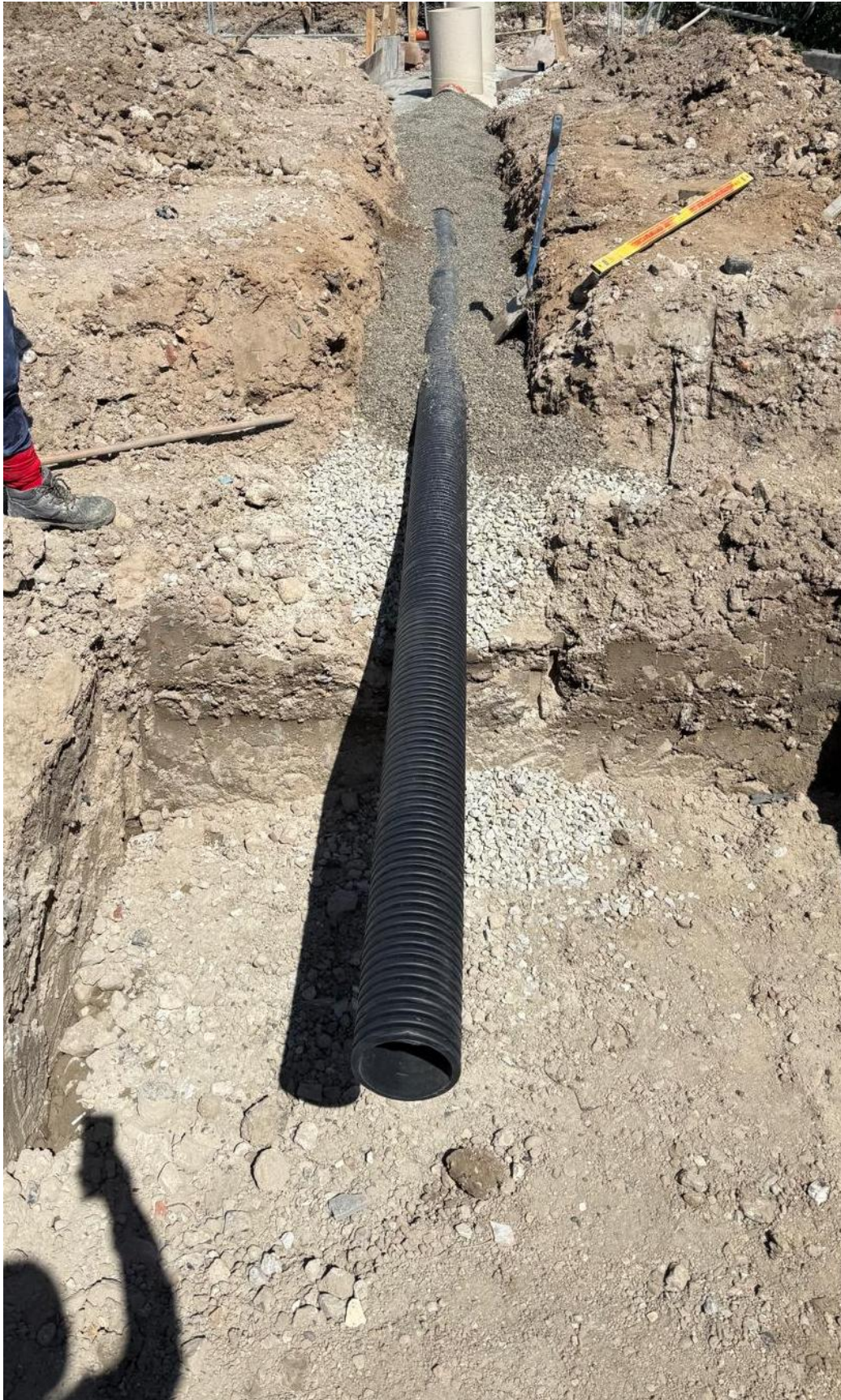
Drain run from interceptor to Hydrobrake – and dig to formation level.
