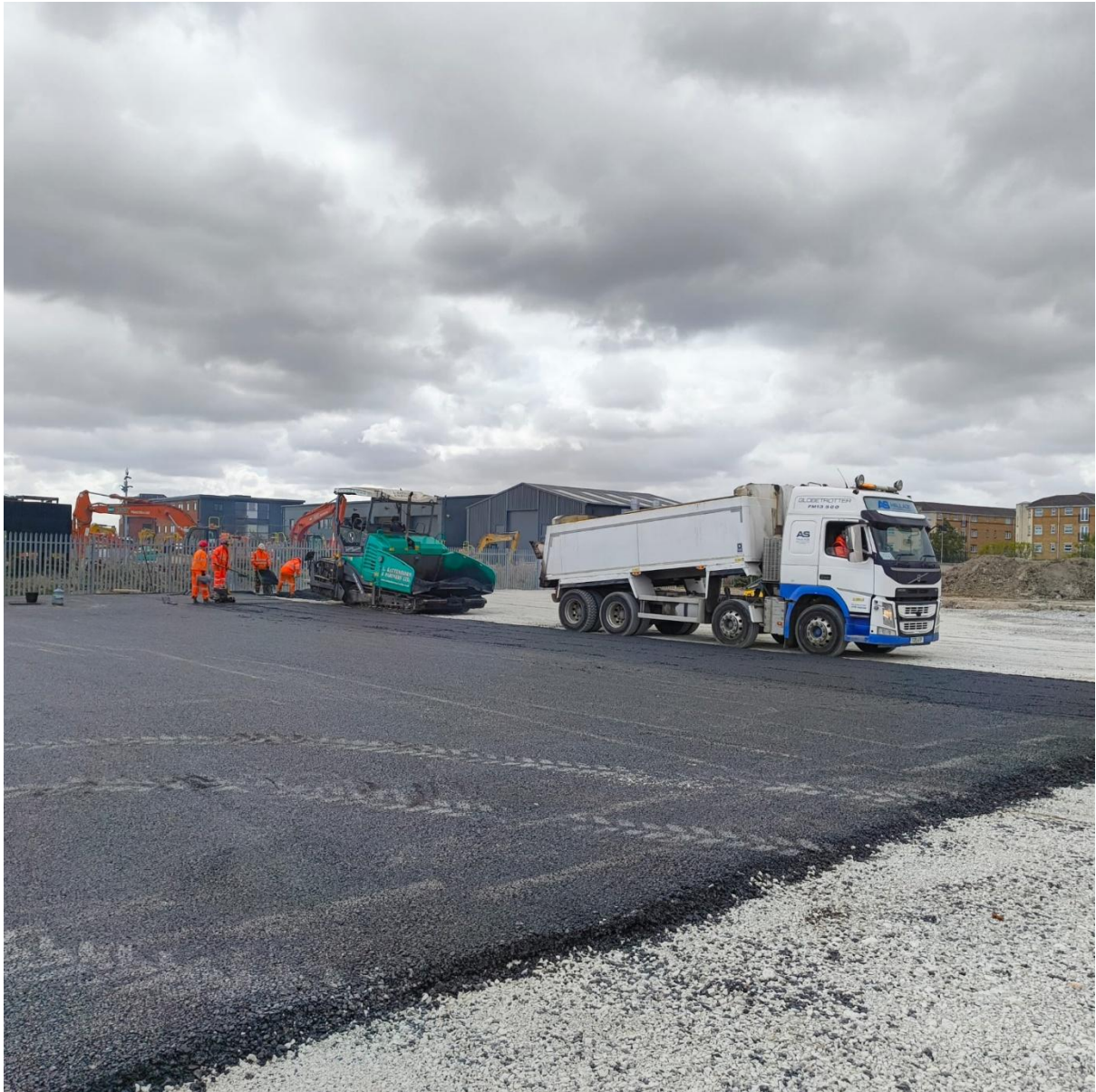
Permeable Tarmac installation
