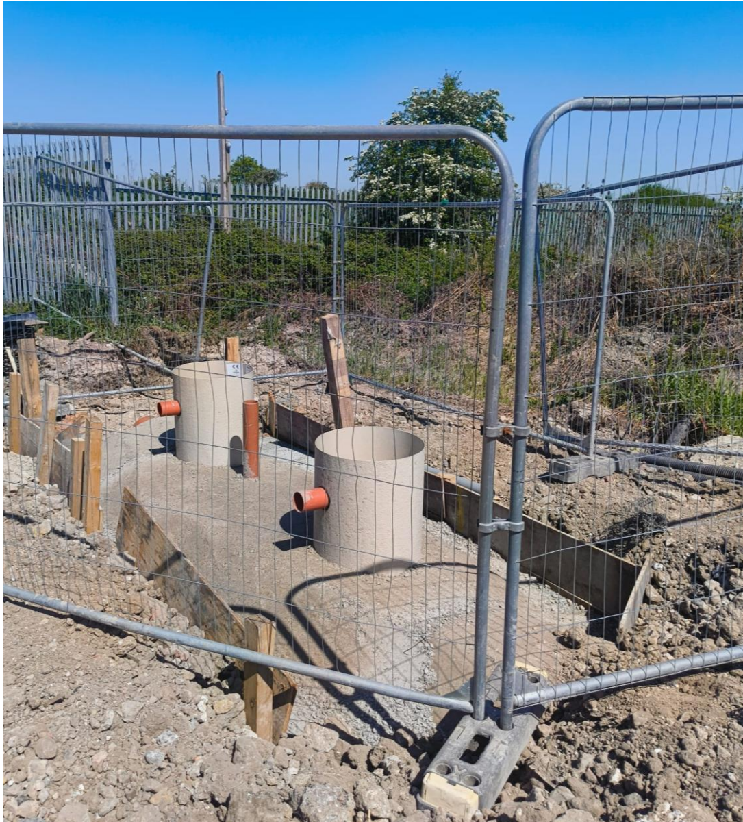
Interceptor backfilled
