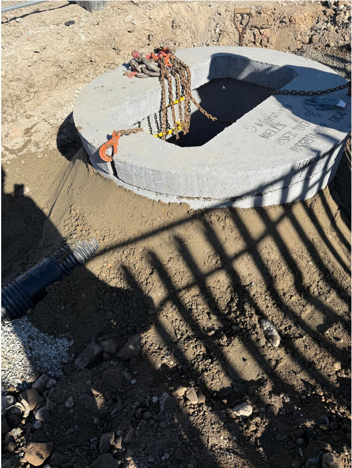
Hydrobrake Construction
