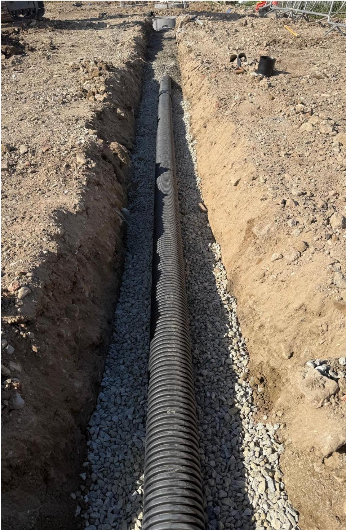
Drainage run from interceptor towards Peravoid / PVOD diffuser unit
