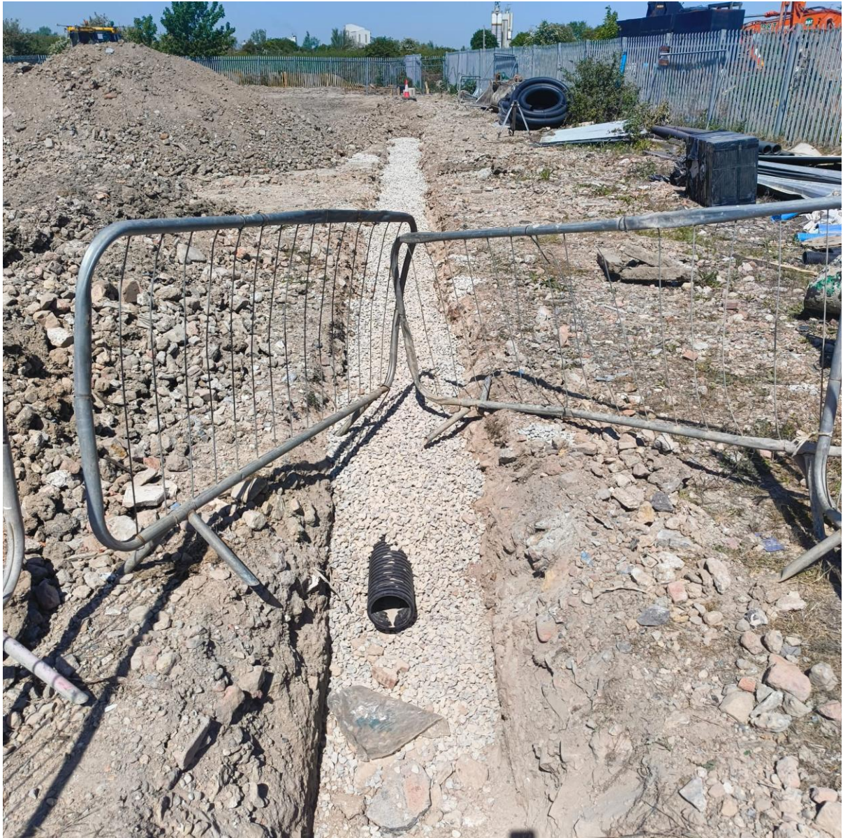
Run backfilling
