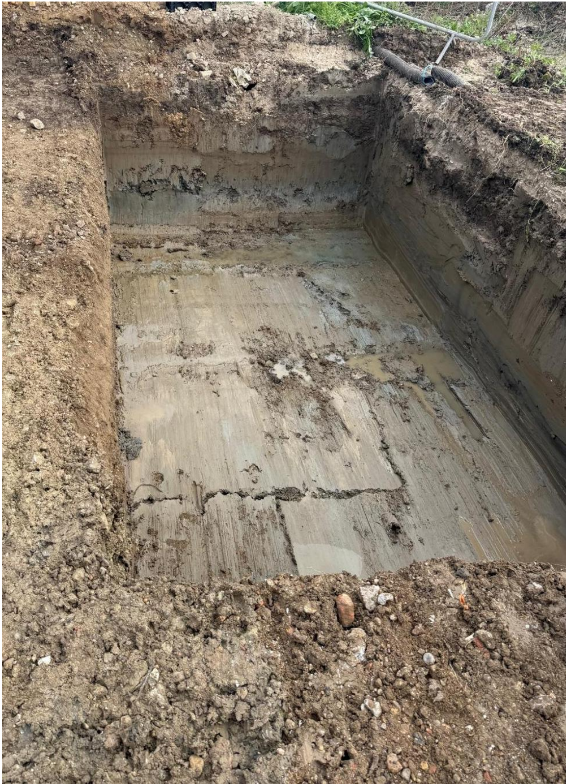
Interceptor excavation to Formation Level.
