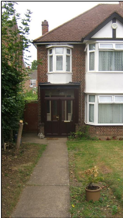
Photo 14 General view of front elevation / roof line
