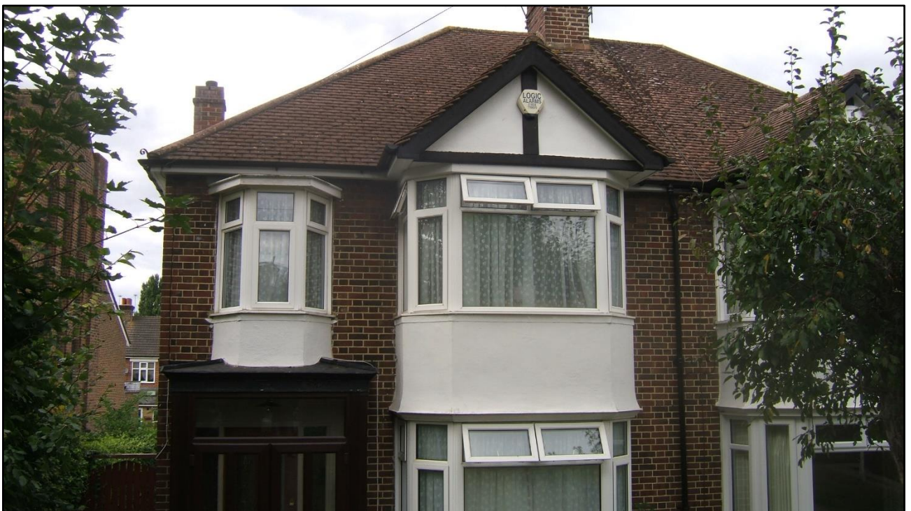
Photo 13 Front elevation view of first and roof level
