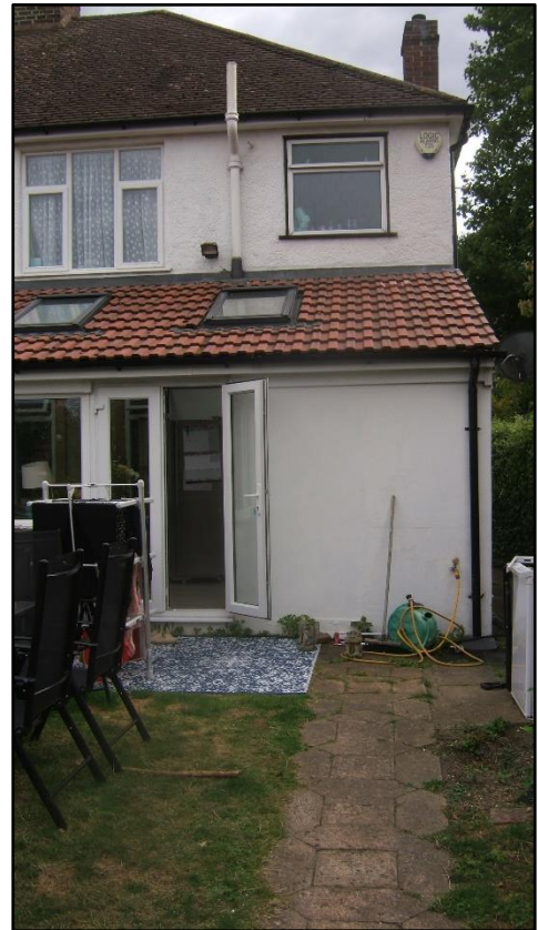
Photo 15 General view of rear elevation / roof line
