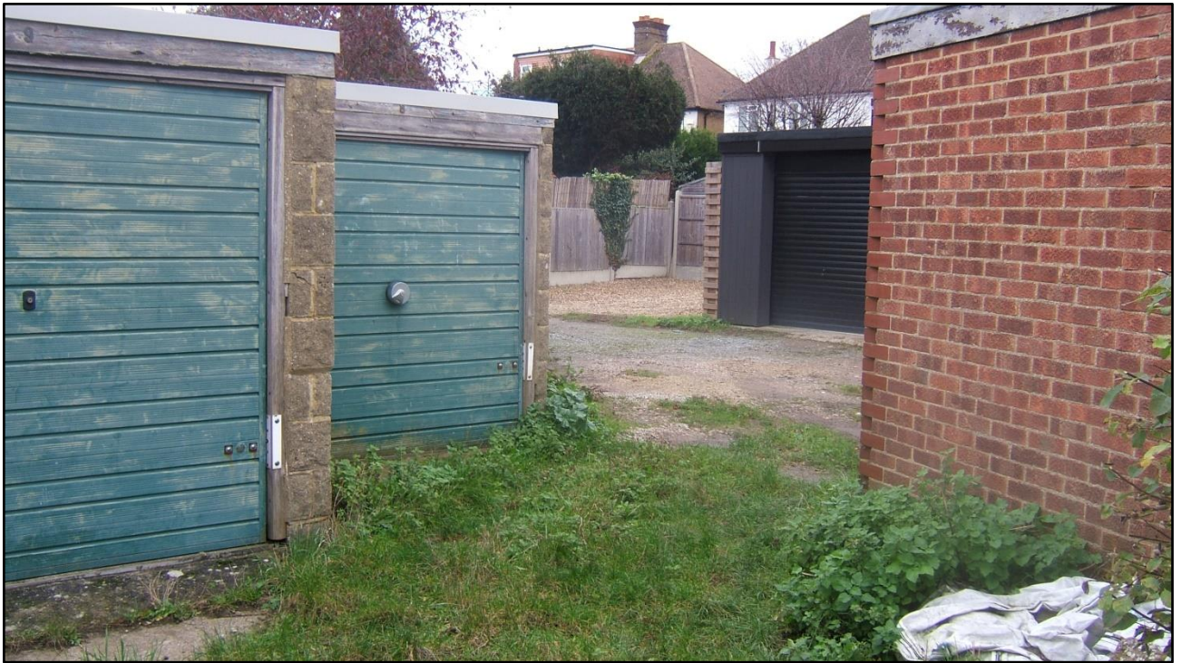
Photo 11 View taken from service road showing restrictive access between existing garages – looking towards access point No 1 from Meadow Road. (Refer to DWG 010 to 030 for location).
