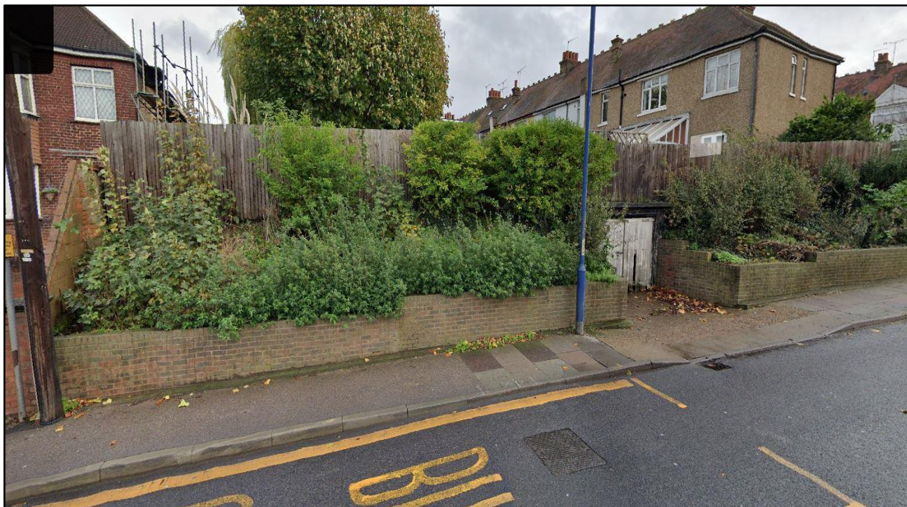
Photo 5 Existing dropped kerb opposite 241 Wrotham Rd / St Mary's Church. NOTE: Telegraph pole to L/H side of photo = telegraph pole as seen in photo 4 (Refer to DWG 010 to 030 for location).
