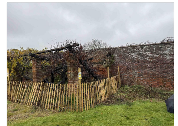
4. VIEW SHOWING COLLAPSED ROOF STRUCTURE
