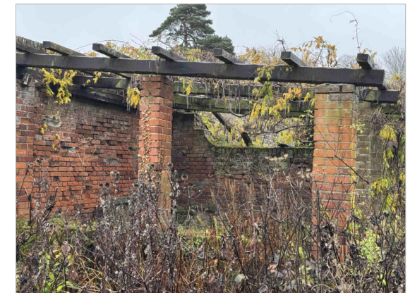
2. VIEW SHOWING CENTRAL DIVIDING BRICK WALL BEHIND PIERS
