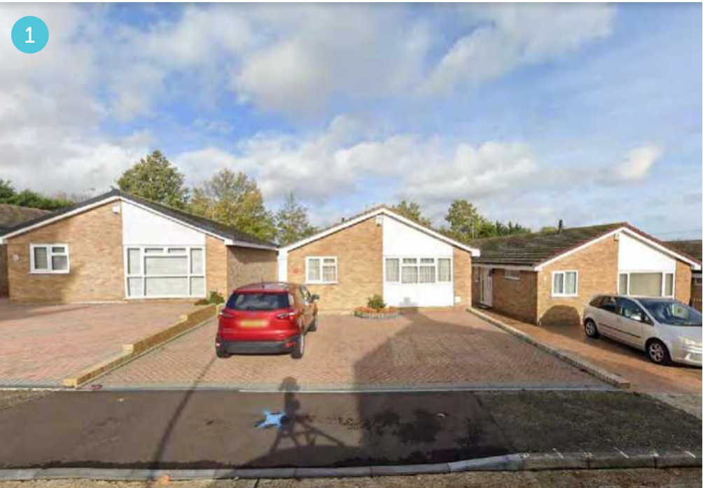
Worchester Close - Shallow Pitches With Light Brickwork
