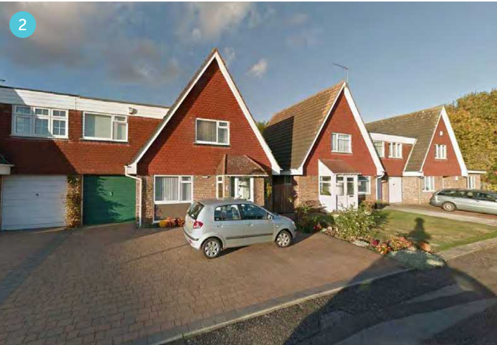
Bramley Close - Prominent Gable Ends With Red Tiles to First Floor and Light Brickwork to Ground
