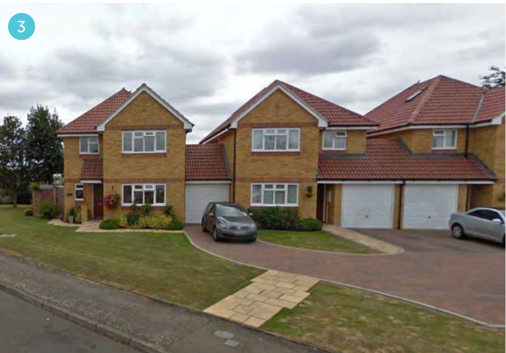
The Drove Way - Prominent Gable Ends & Horizontal Brick Soldier Course Banding
