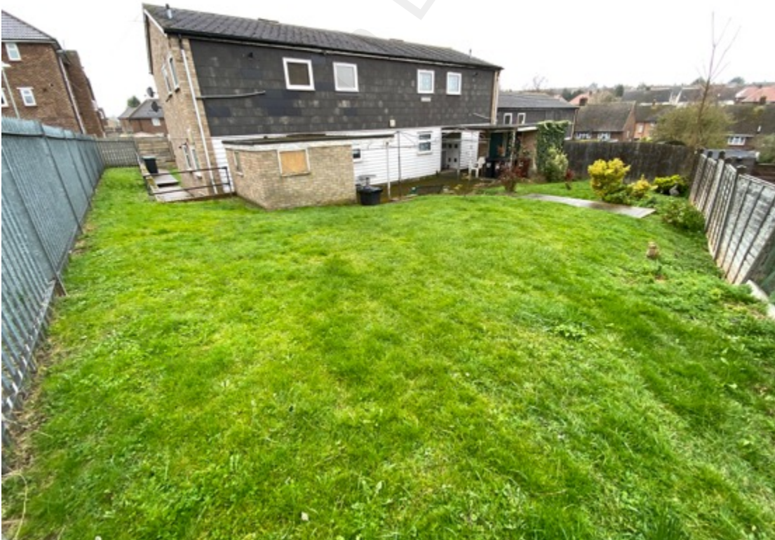
Photograph 4: View of buildings 28-34 and 36-42, rear aspects looking south-west
