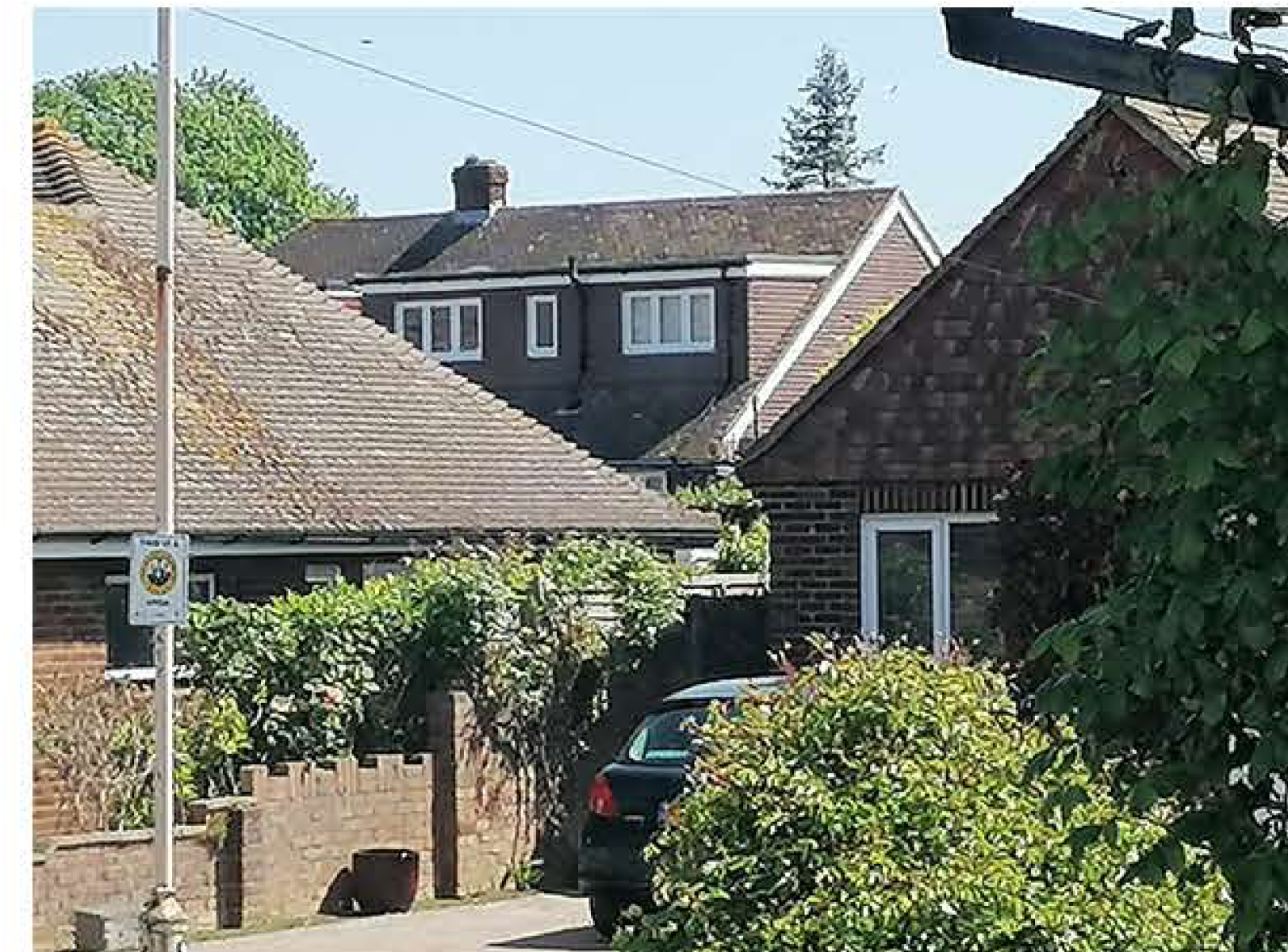
PICKWICK GARDENS, NORTHFLEET - REAR VIEW REAR DORMER SEEN FROM PEPY'S CLOSE
