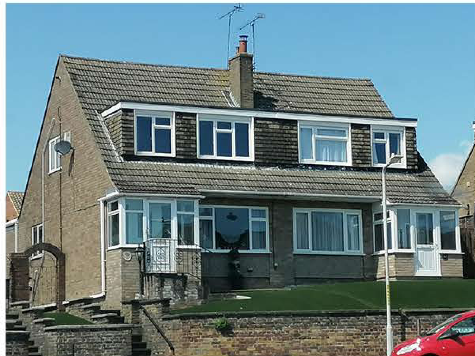
PAINTER'S ASH LANE, NORTHFLEET - STREET VIEW FRONT DORMER
