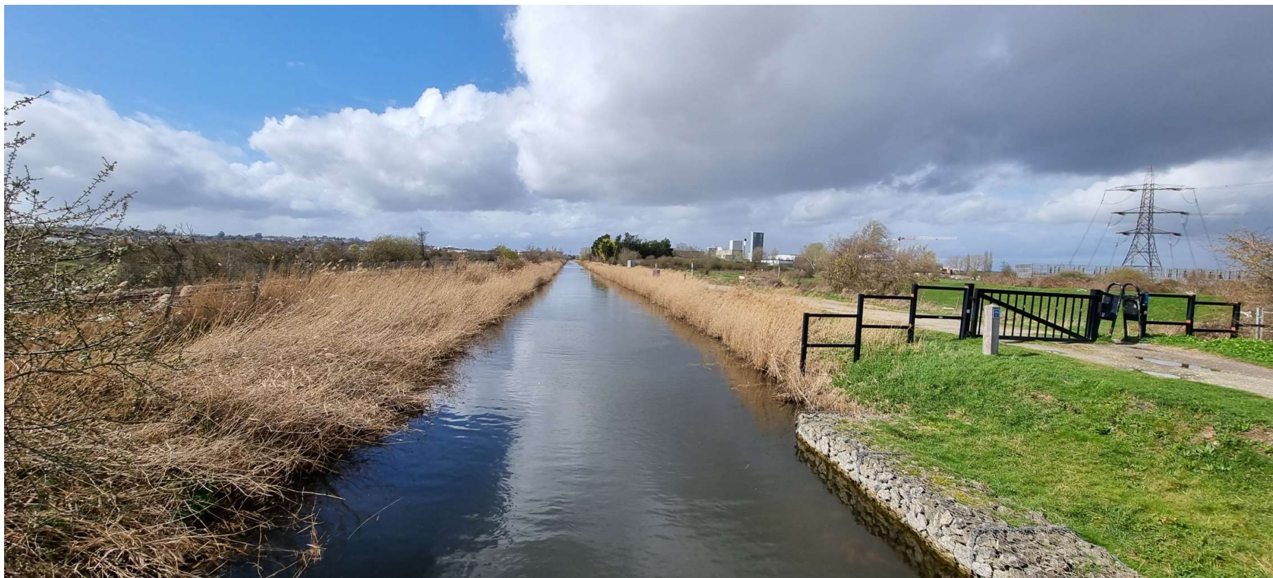
Plate 8: A view northwest along the Thames and Medway Canal from swing bridge (TQ 67 SE 49)
