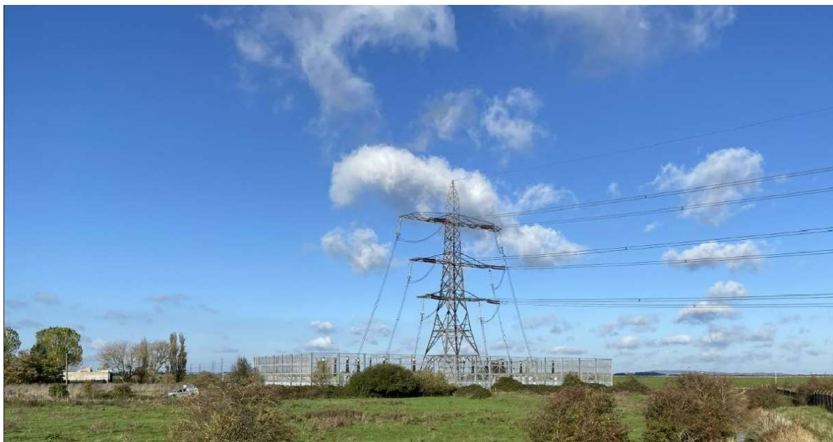
Photo 3 Existing Tilbury Tunnel Headhouse and SEC.
