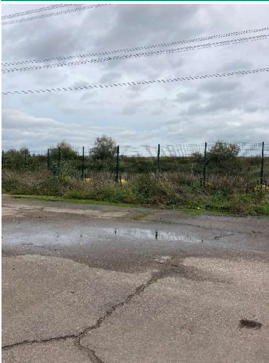
Photograph 3 – Hardstanding at Tilbury Site
