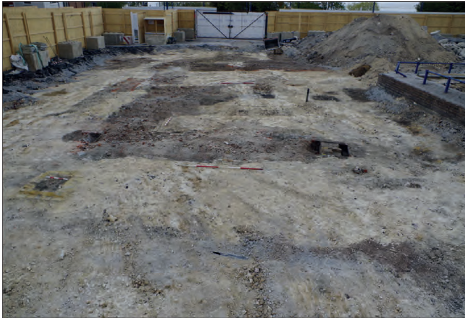
Plate 7: Irregular basement foundation 1240, viewed from the south
