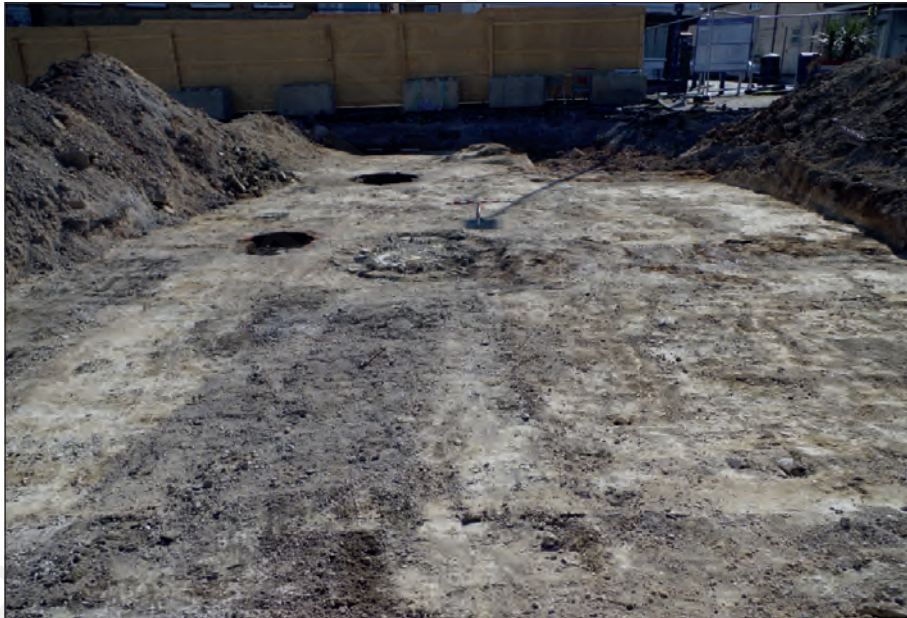
Plate 20: Wells/cess pits 1025, 1026 and 1027, viewed from the west
