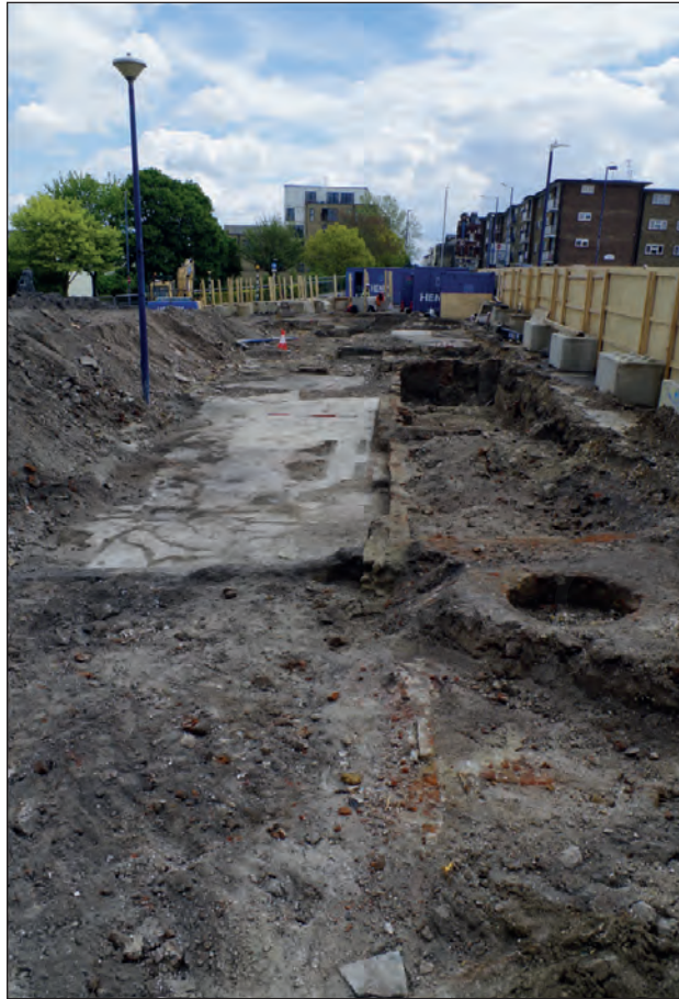
Plate 5: Terraced building 1239, viewed from the west
